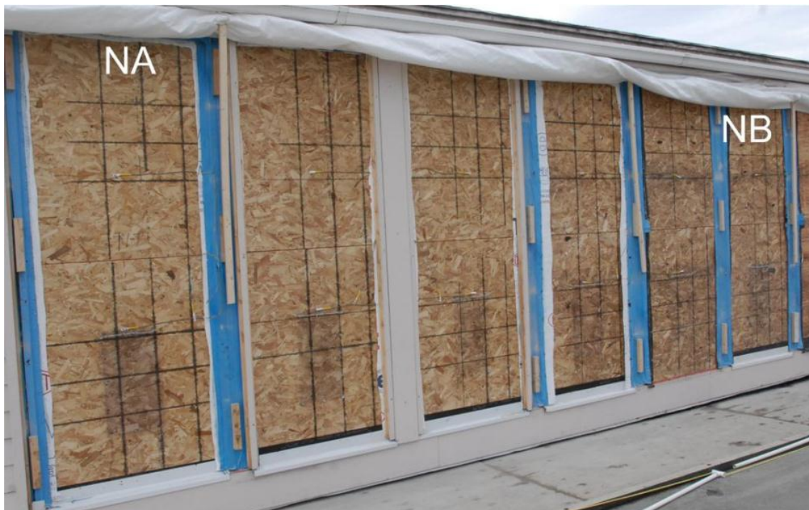
Figure 46. Exterior OSB sheathing on the north orientation immediately following deconstruction
