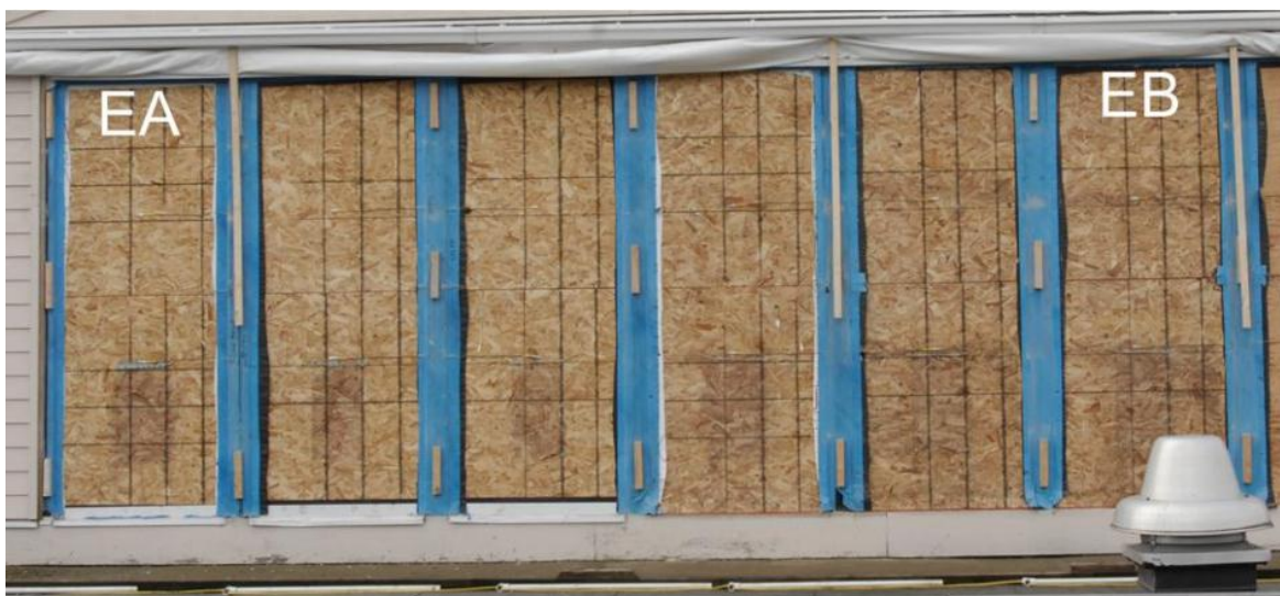
Figure 48. Exterior OSB sheathing on the east orientation immediately following deconstruction
