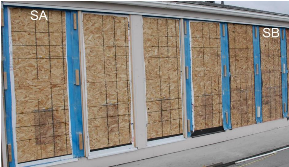
Figure 49. Exterior OSB sheathing on the south orientation immediately following deconstruction
