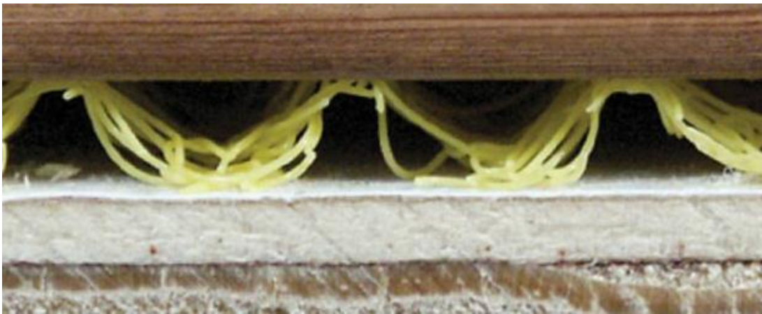
Figure 18. Example of drainage mesh between two sheet materials
