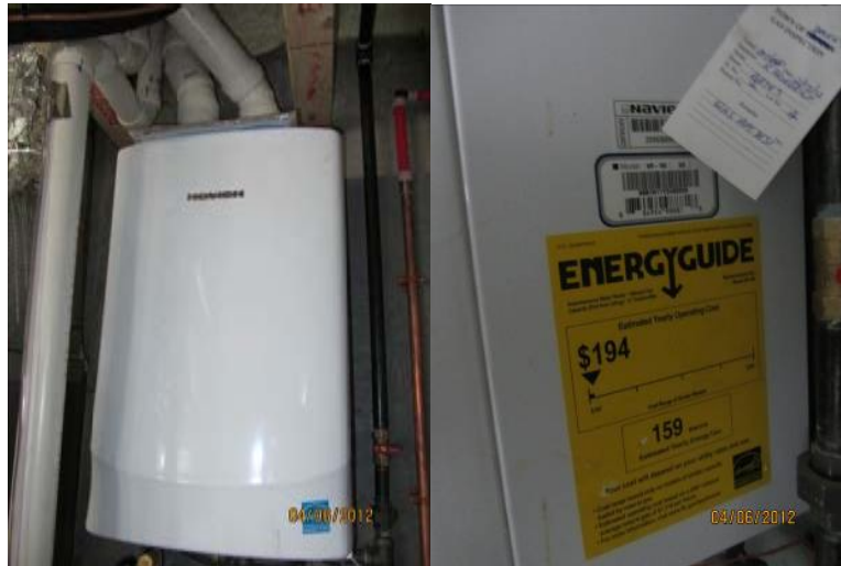
Figure 13. Tankless water heater
