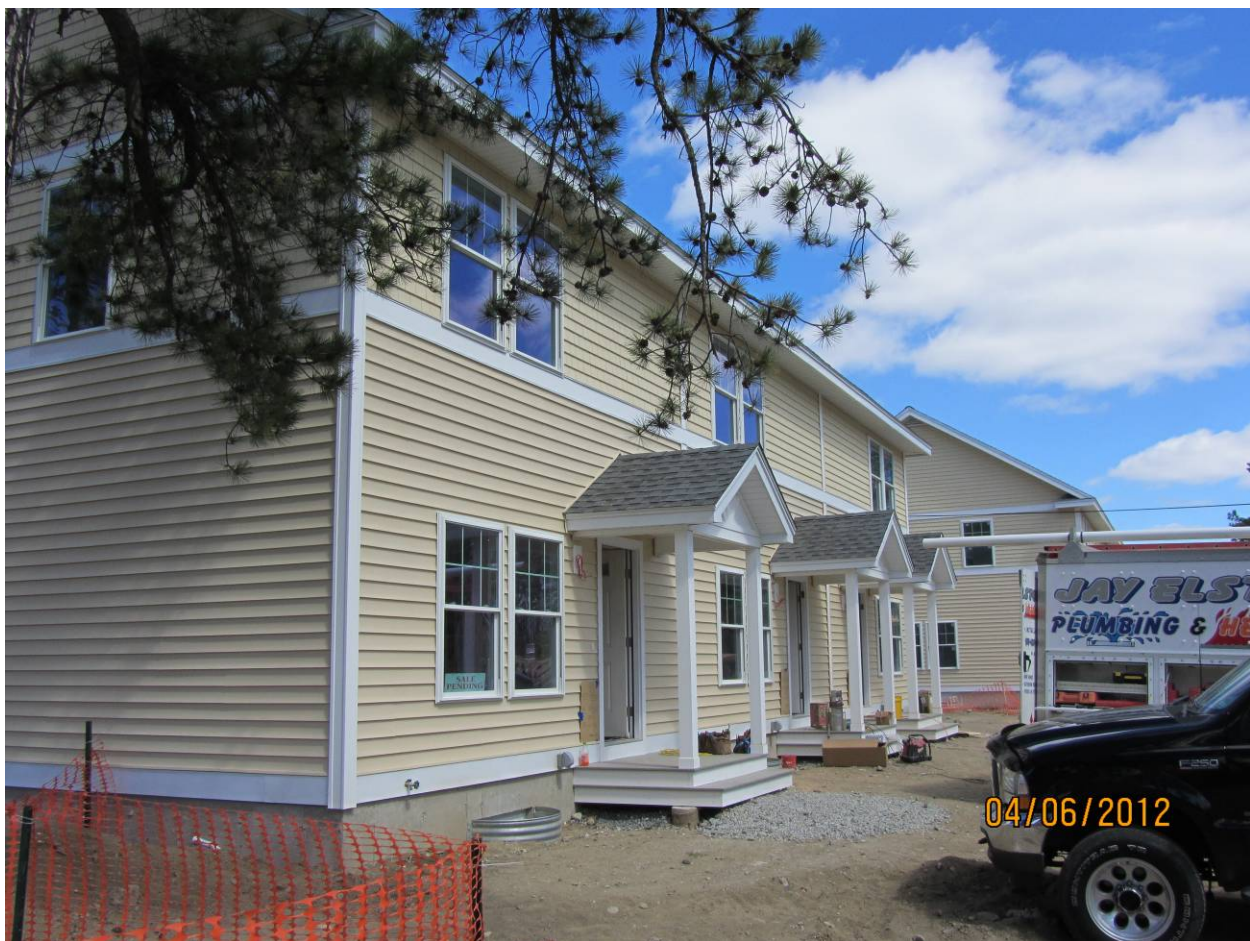
Figure 2. Photo of the prototype triplex nearing completion
