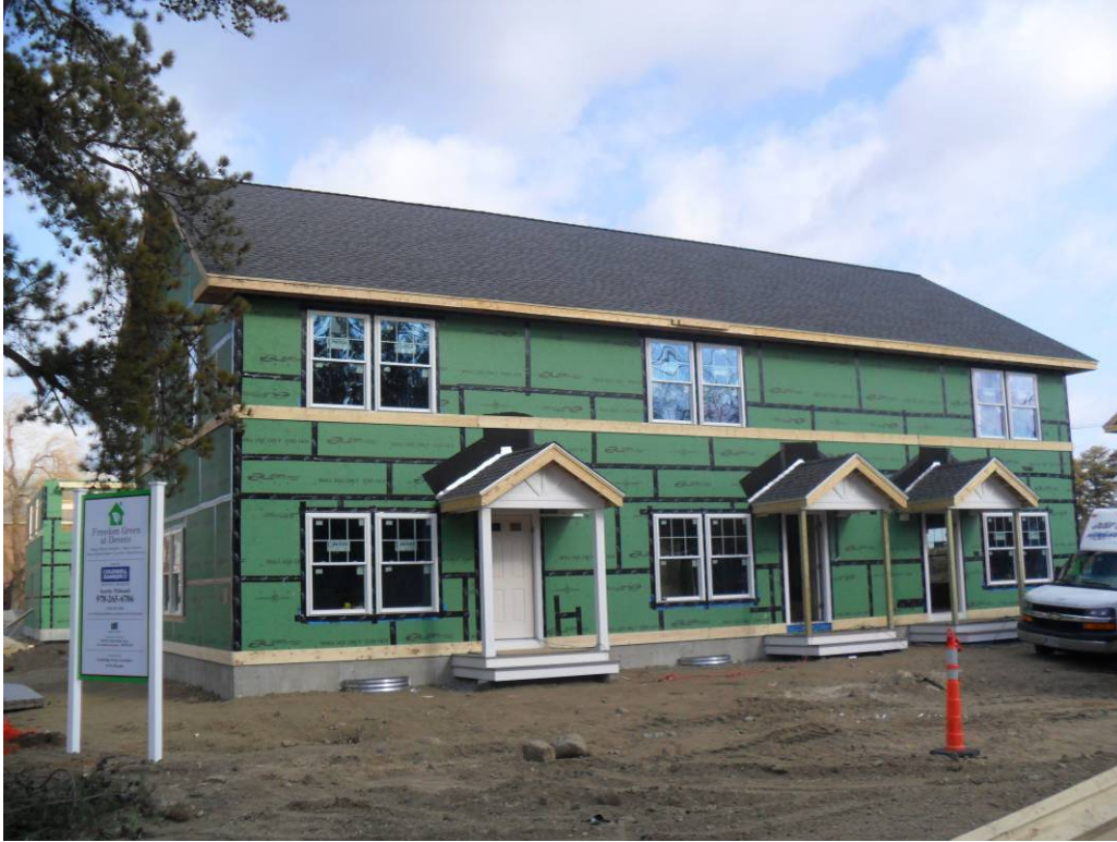
Figure 6. Triplex during construction
