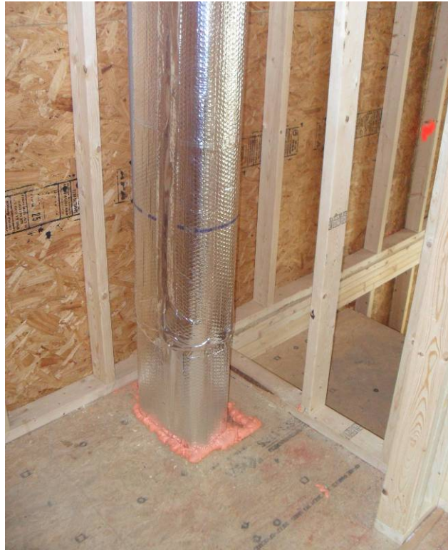
Figure 11. Duct during framing
