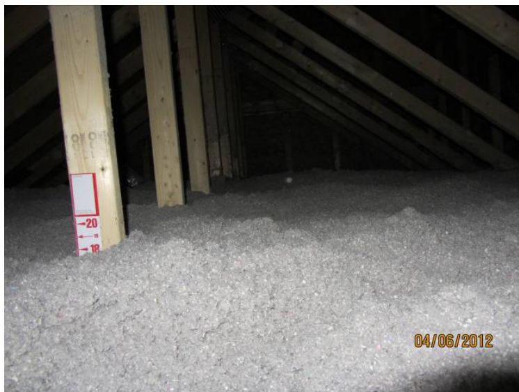
Figure 9. Attic insulation
