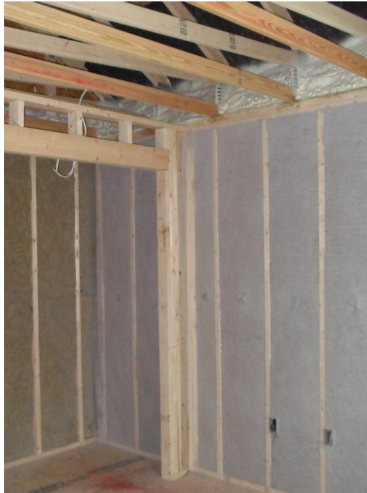
Figure 7. Above-grade walls with dense pack cellulose insulation
