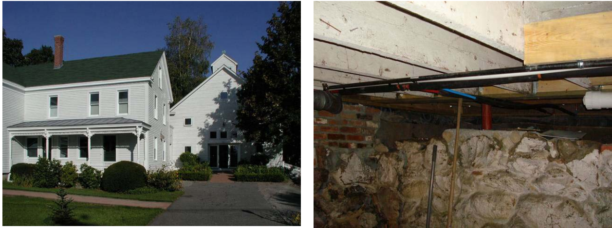
Figure 18. Overview of Westford House/Barn, existing foundation conditions (Lstiburek 2010a)
