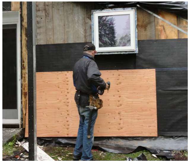
Figure 47. Westford House/Barn recladding and sill beam inspection
