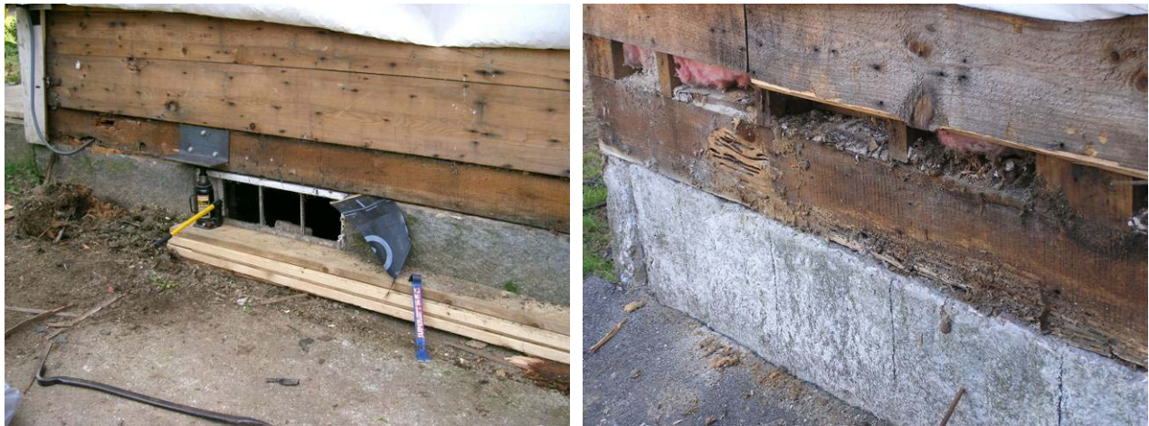
Figure 42. Sill lift and pre-retrofit sill beam condition at Bedford Farmhouse
