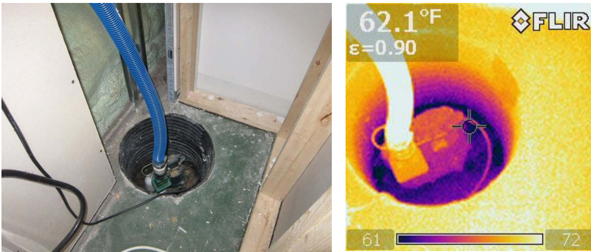
Figure 56. Sump pit temperatures, Concord House
