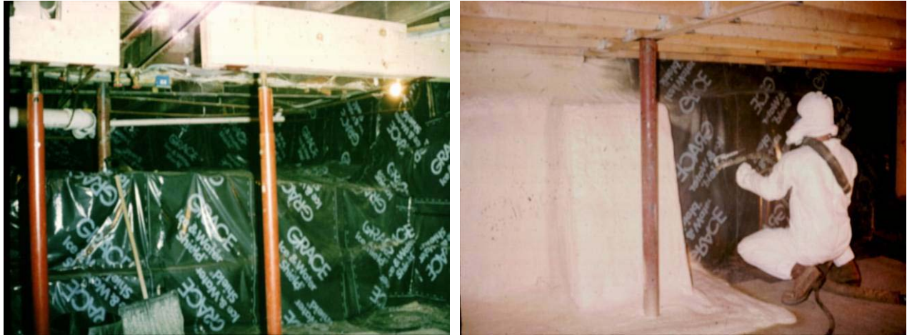
Figure 20. Self-adhered membrane and spray foam installation (Lstiburek 2010a)
