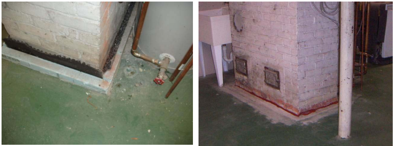
Figure 30. Drainage mat penetration at chimney; retrofit sealing of drainage mat
