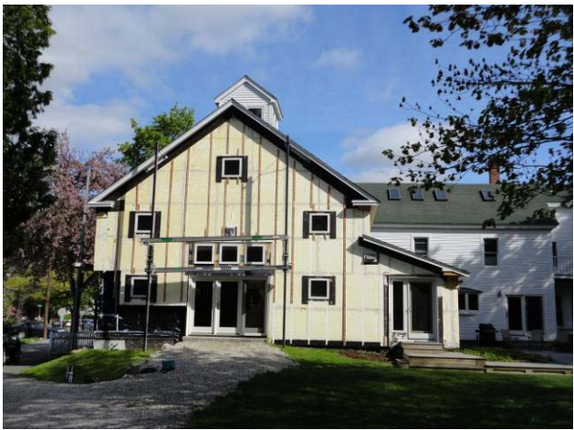
Figure 47. Westford House/Barn recladding and sill beam inspection
