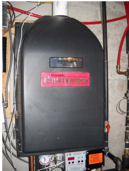
Figure 5. Wall hung condensing boiler
