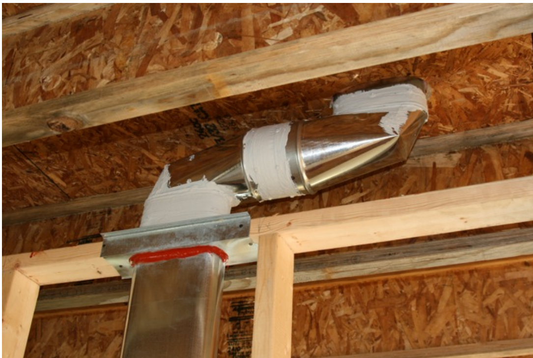
Figure 16. Typical duct sealing at boot and through interior partition top plate
