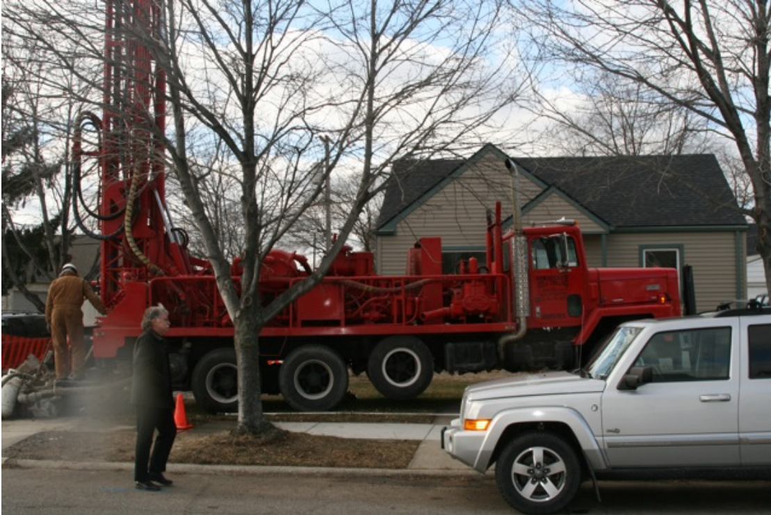
Figure 1. Photograph of a well borehole operation for a GSHP system in the NSP2 neighborhood
