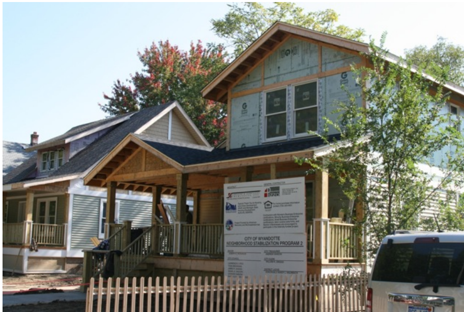
Figure 3. Wyandotte NSP2 houses (Walnut 1 and 2) under construction
