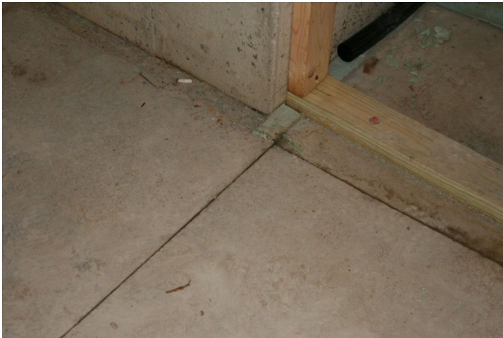
Figure 12. Photograph of slab edge insulation
