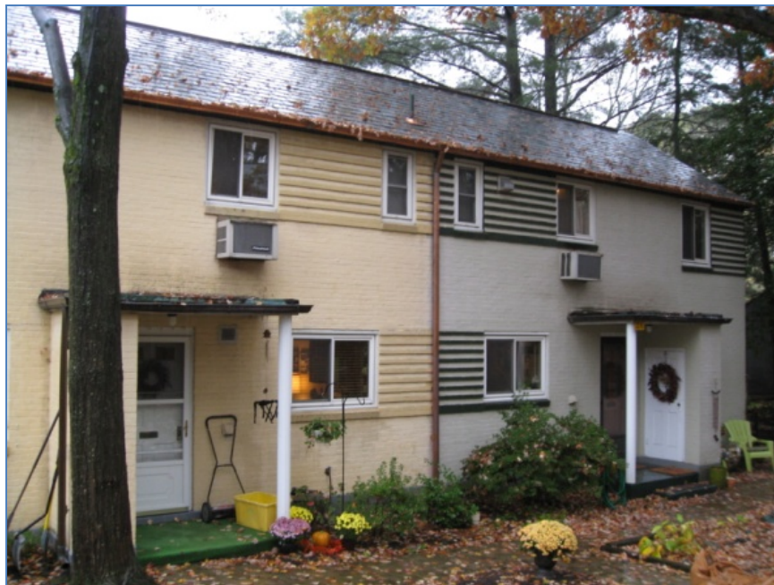
Figure 3. Wood frame brick building, front elevation, two units.
