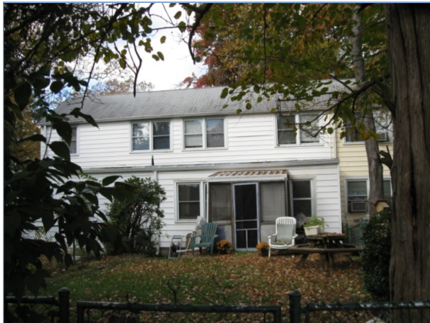
Figure 6. Wood frame vinyl building, rear elevation, three units.
