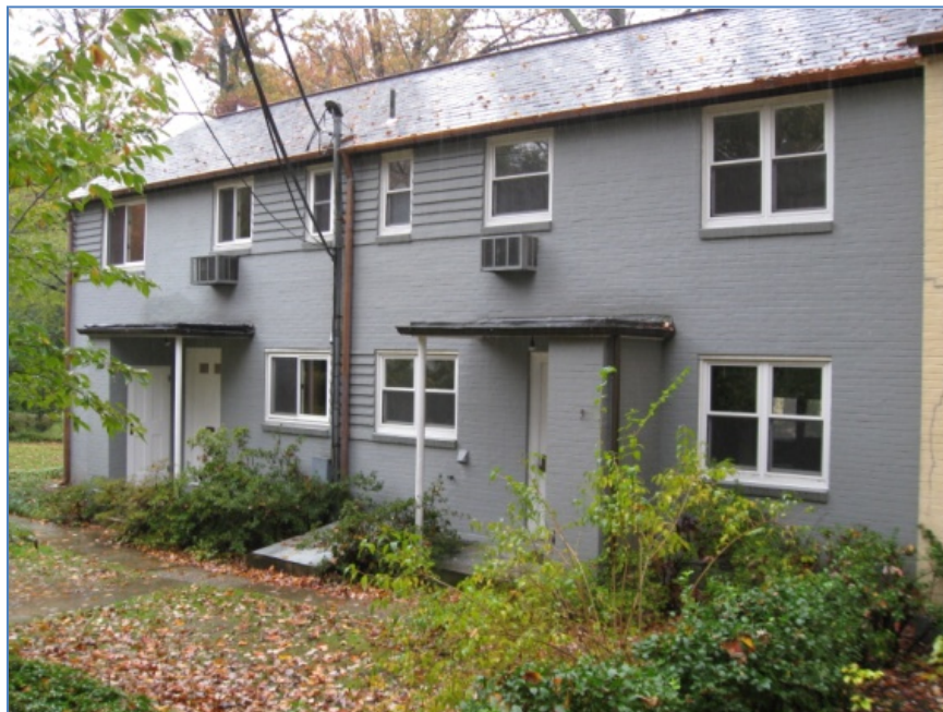
Figure 4. Wood frame brick building, front elevation, two units.
