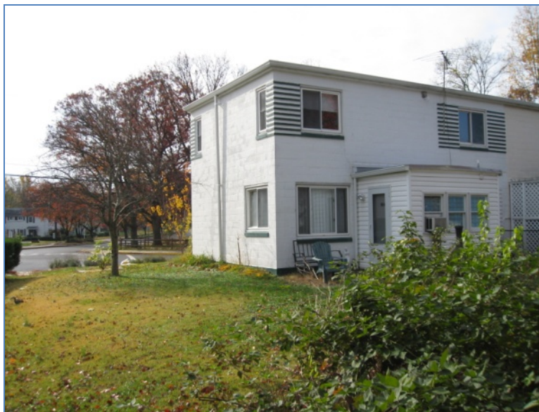
Figure 2. Block building, one end unit, rear.
