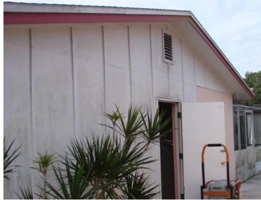
Figure 12. Typical shallow roof pitch of Florida homes built before 1980
