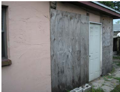
Figure 33. Pre-retrofit exterior wall of porch converted into conditioned space
