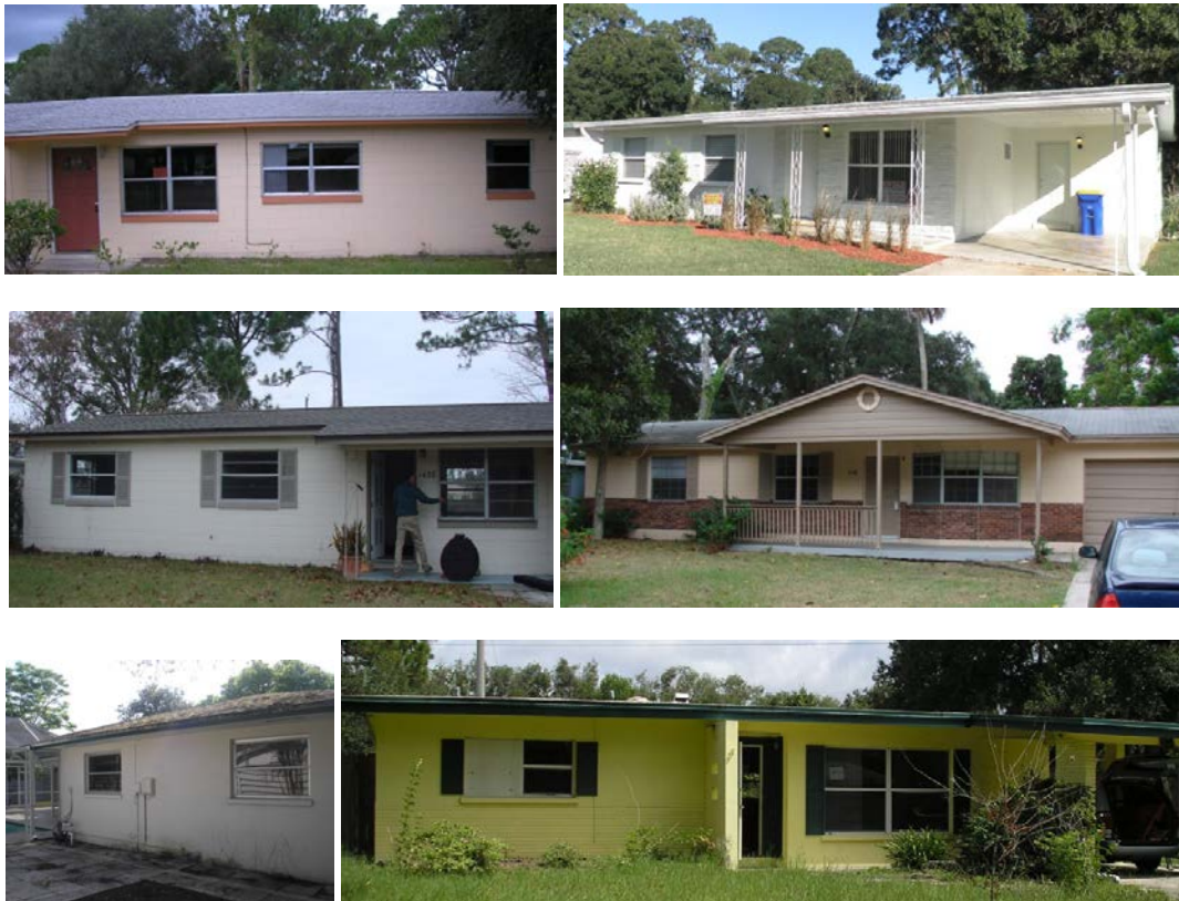
Figure 5. Study homes of typical character with ranch style floor plans, slab-on-grade foundations, concrete block exterior walls, low sloped roofs, and 8-ft ceiling heights
