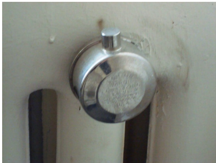
Figure 11. Gorton No. 4 angle radiator vent. Gorton models are made in No. 4, 5, 6, C, and D, ranging from 4 with the smallest orifice (for warm apartments) to D with the largest (for cool apartments)
