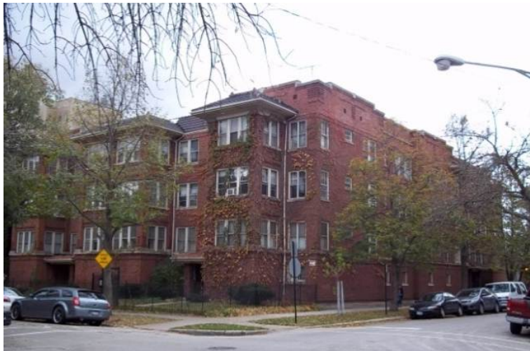
Figure 1: Typical brick three-story walk-up in Chicago. This building type commonly has a steam system and can be out of balance.
