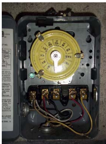
Figure 9. Time clock control for a steam boiler (used with permission from CNT Energy 2011)
