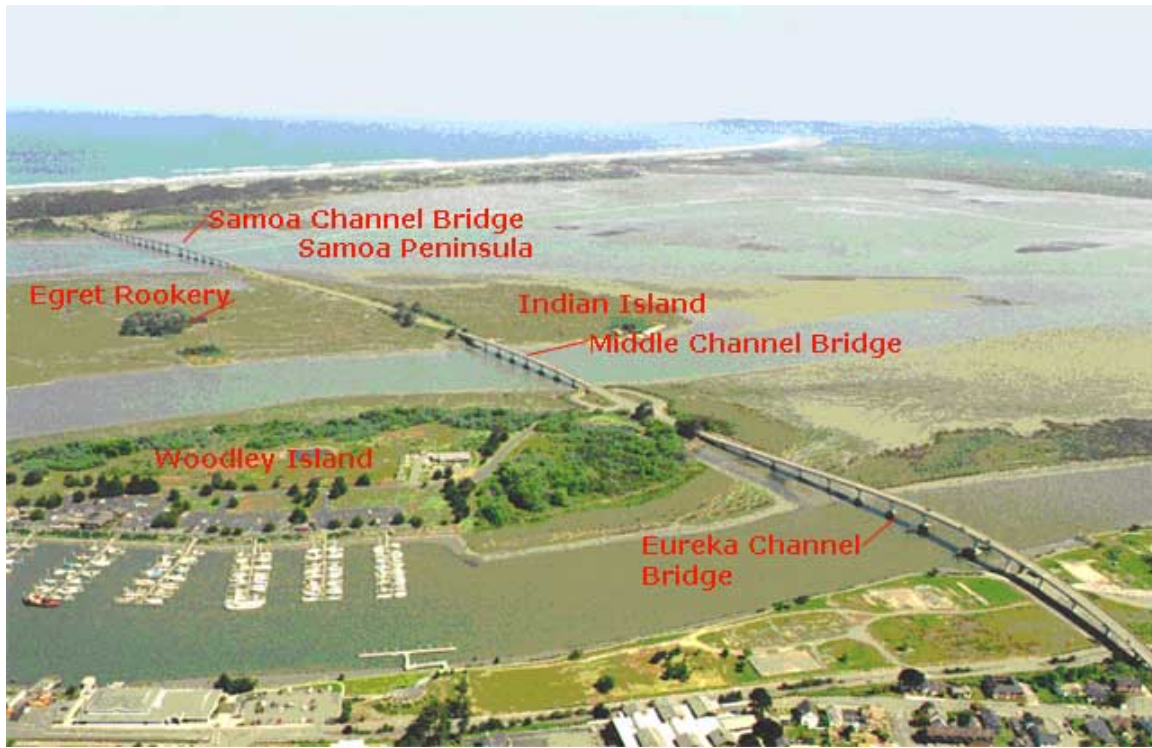
Figure 3. Humboldt Bay channel bridges (courtesy of Caltrans)
