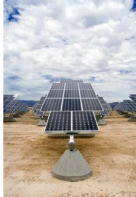
Source: NREL PIX 15280
