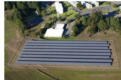
Source: NREL PIX 17395
