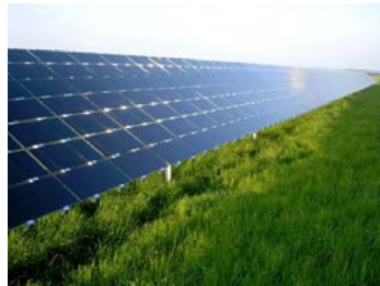
Source: NREL PIX 14726
