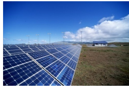
Source: NREL PIX-13823
