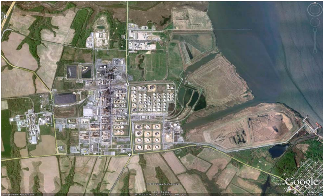
Air Liquide Chemical Plant, DE
