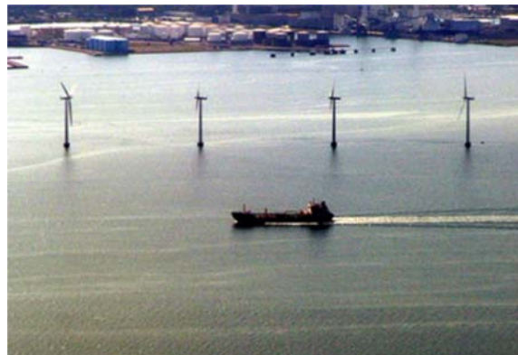
Figure 1-1 Near-shore wind plant in Denmark - produces electricity and serves as aids to navigation
