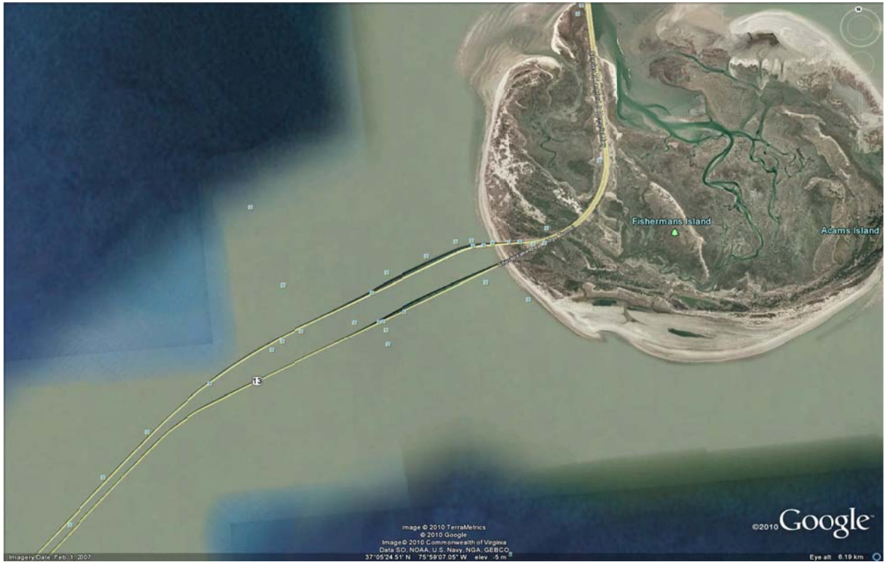
North end, Chesapeake Bay Bridge tunnel
