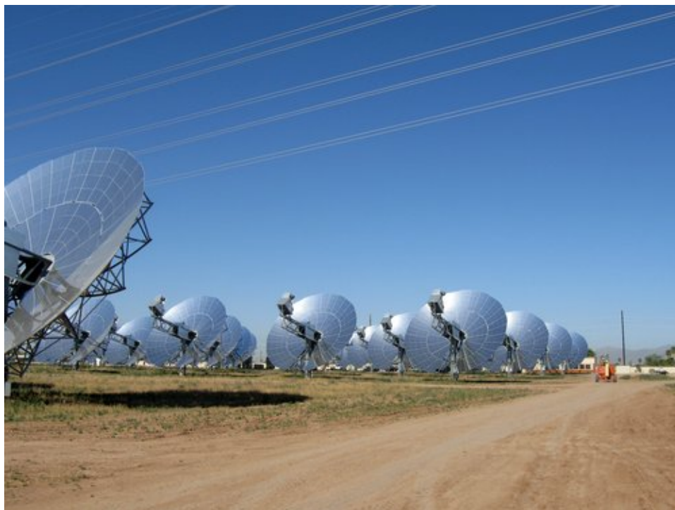
Figure 2-9. 1.5-MW Maricopa, Arizona, solar power plant—60 25-kW dish Stirling systems. Photo by David Hicks, NREL 18379
