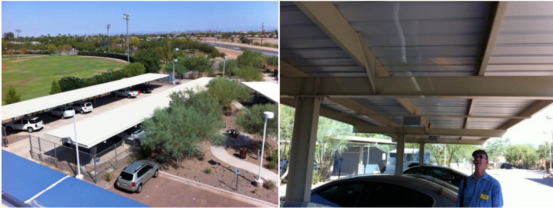
Figure 5-12. Northwest carports looking northwest (left) and carport structure, which would require the attachment of PV support racking (right). Photos by Otto VanGeet, NREL
