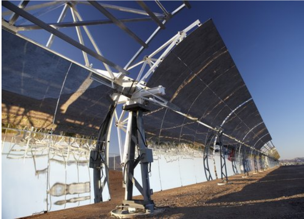
Figure 2-5. Solar trough at a 50 MW plant. Photo by Geri Kodey, NREL 14390
