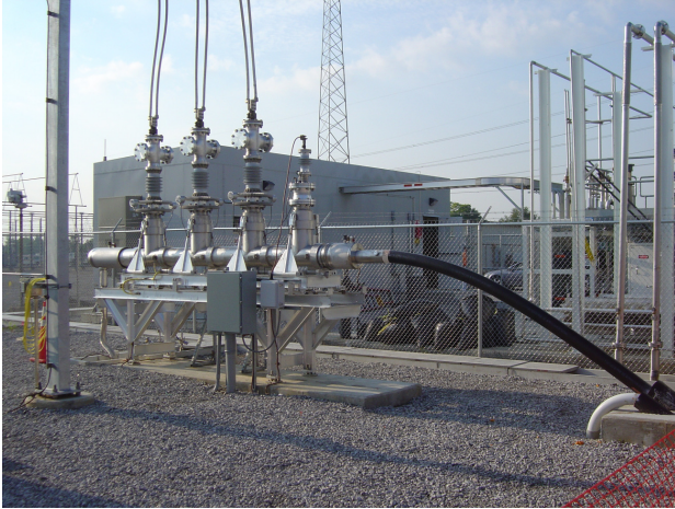
Figure 2. HTS Triax™ Termination
