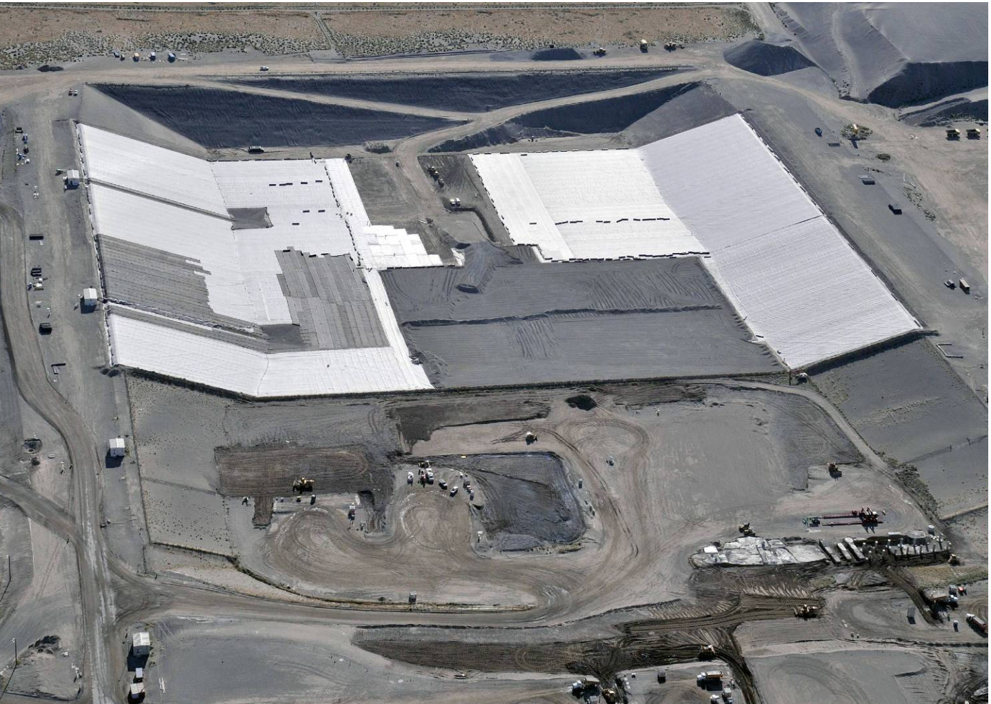
Figure 8. WCH Constructed Super Cells 9 and 10 Simultaneously, Saving Time and Construction Costs.
