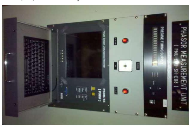
Figure 56: Phasor Measurement Unit (PMU) Installed at IIT's Stuart Building
