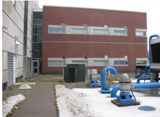
Figure 14. Digital image of the building
