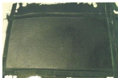
(b) First coating pass (dry)
