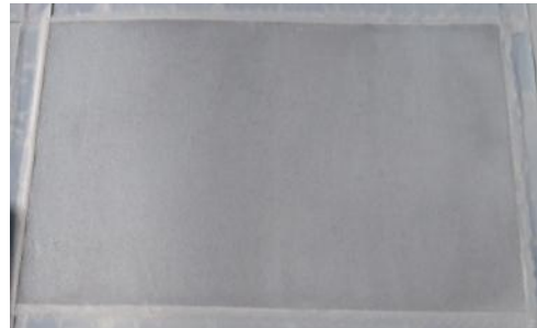
(b) First coating pass (dry)
