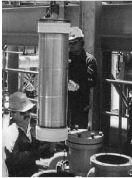
Figure – 1 Commercial CO 2 removal element, pipe and flange housing assembly.
