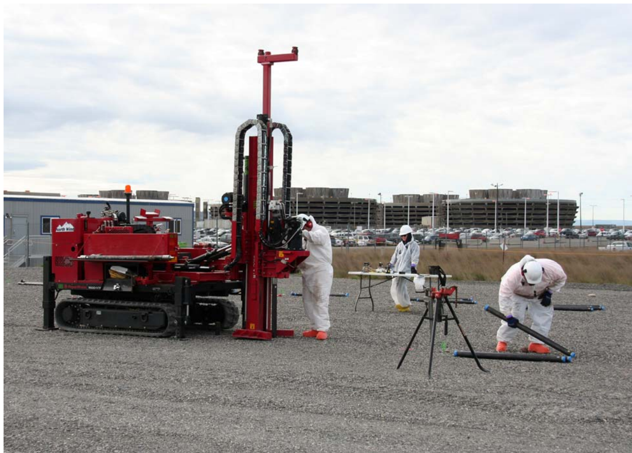
Figure 2. Installation of the Cone Penetrometers at the 618-11 Burial Ground.
