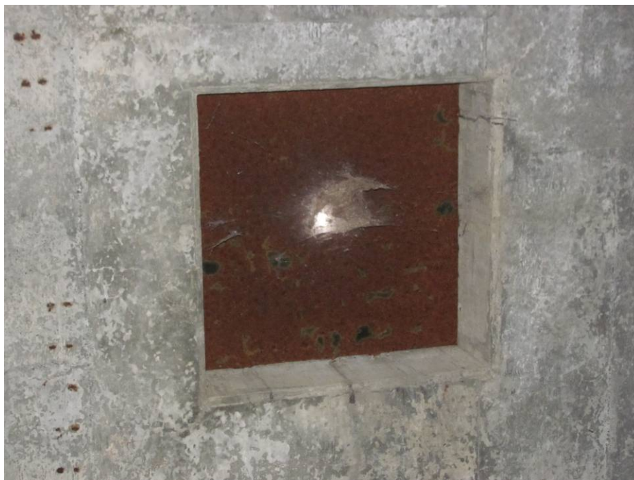
Figure 6. Typical Clearwell Hatch Cover (no urine staining observed).
