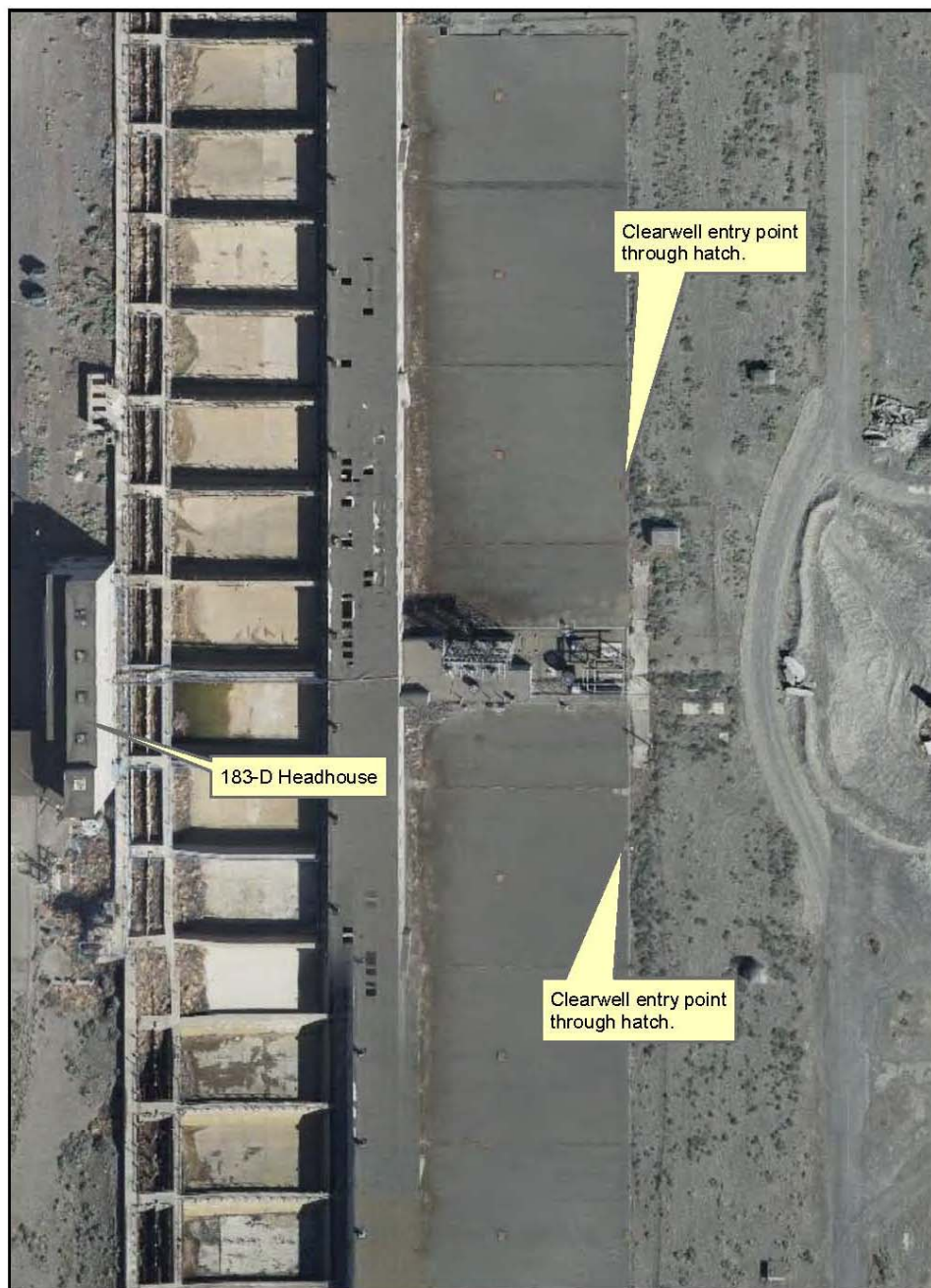
Figure 3. 183-D Clearwell Personnel Entry Points.
