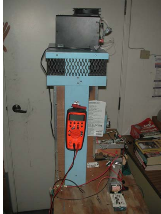
Figure 35. Power Conditioning Unit (PCU) Bench Test
