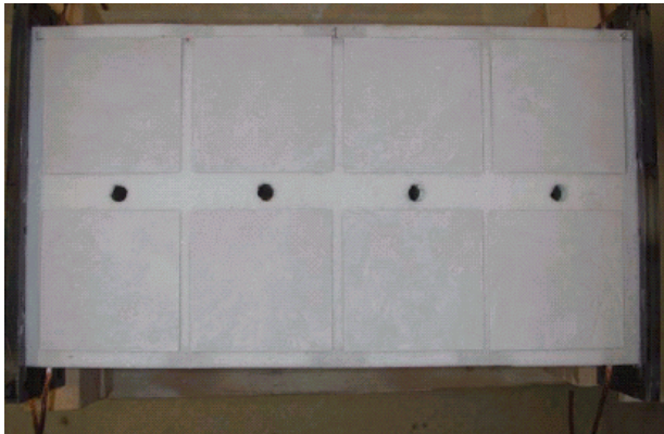
Figure 30. Additional Insulation Installed
