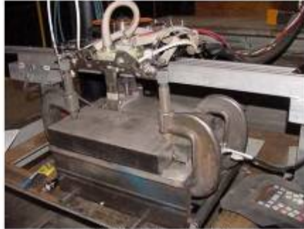
(a) Clamping of joint
