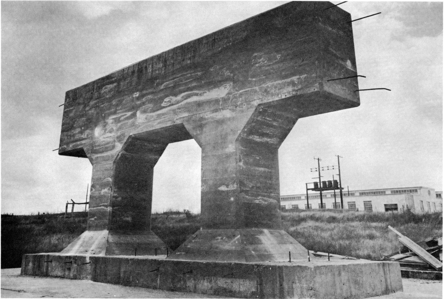
North side and west end of bridge pier
