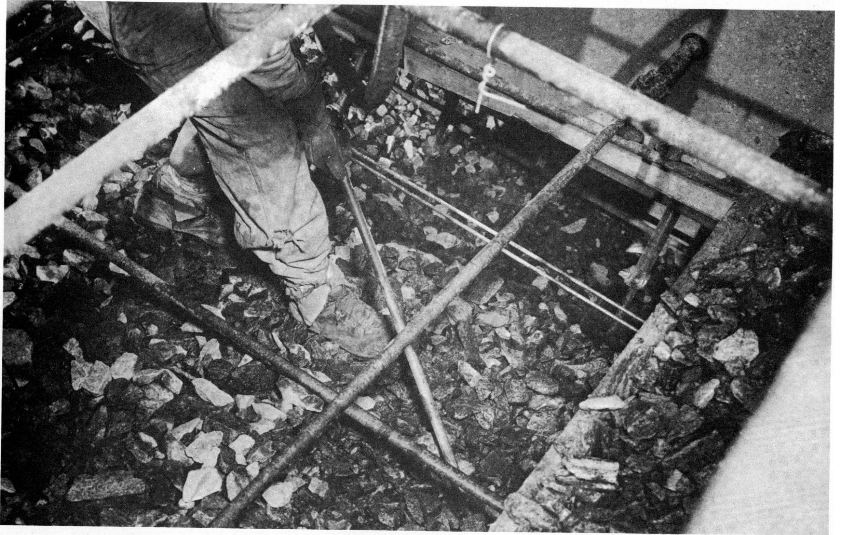
Placing coarse aggregate under blockout with compressed air jet
