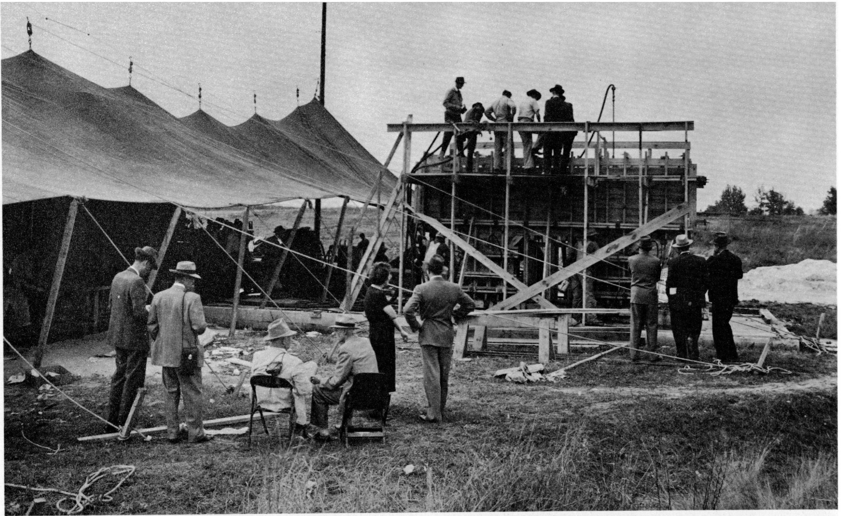
Grouting bridge pier. Tent-covered block and equipment for batching, mixing and placing to left
