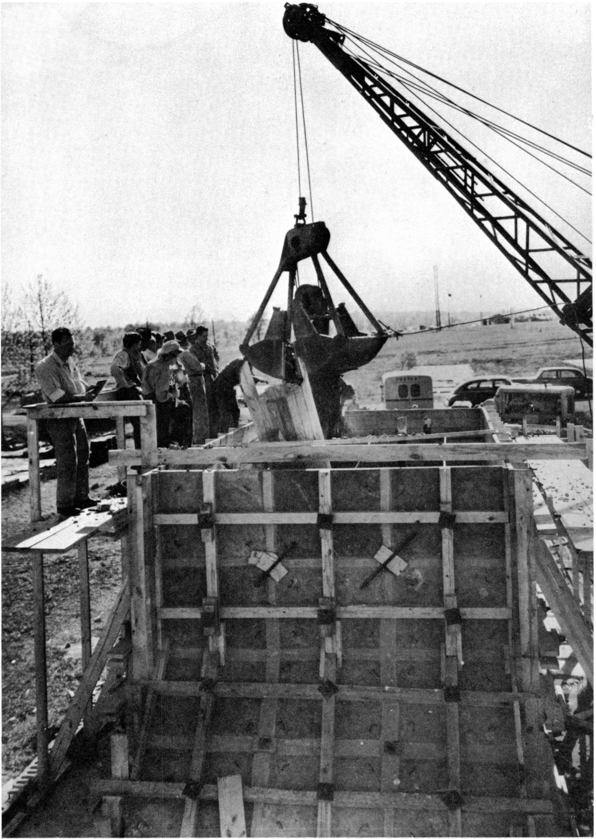
Placing aggregate in test block
