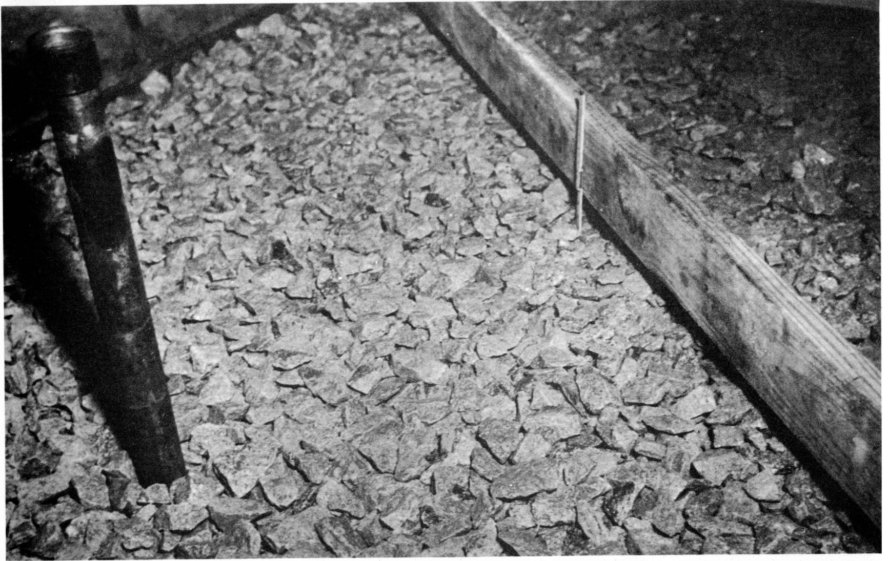
Test block after coarse aggregate placement
