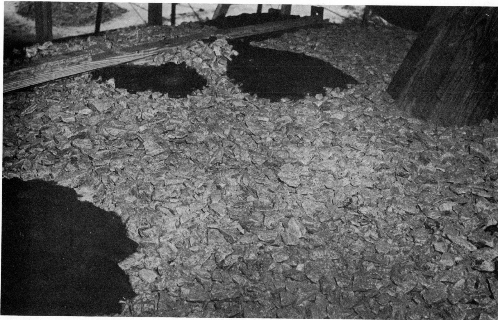
Grout eruption through coarse aggregate
