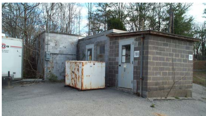
Fig. 2. Pilot Pit Facility.
