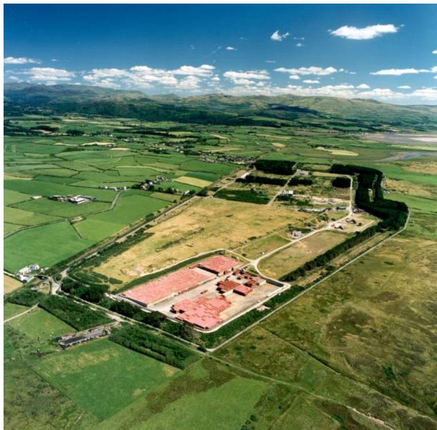
Fig. 1. Aerial View of the BNFL Drigg Site
