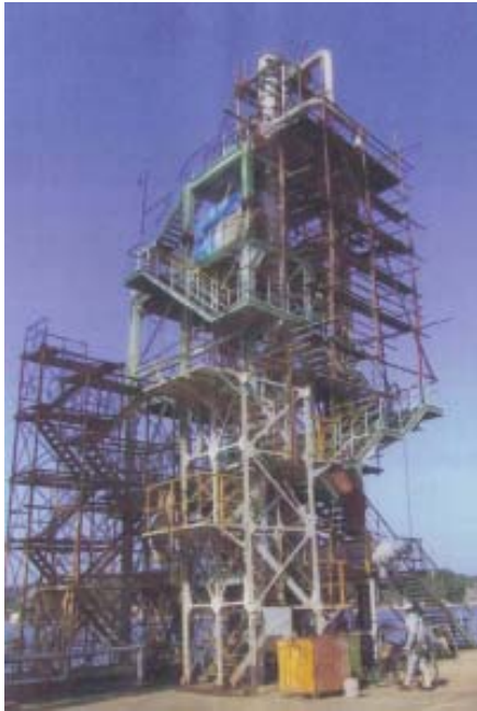
Fig. 7. Facility for Experimental Study
