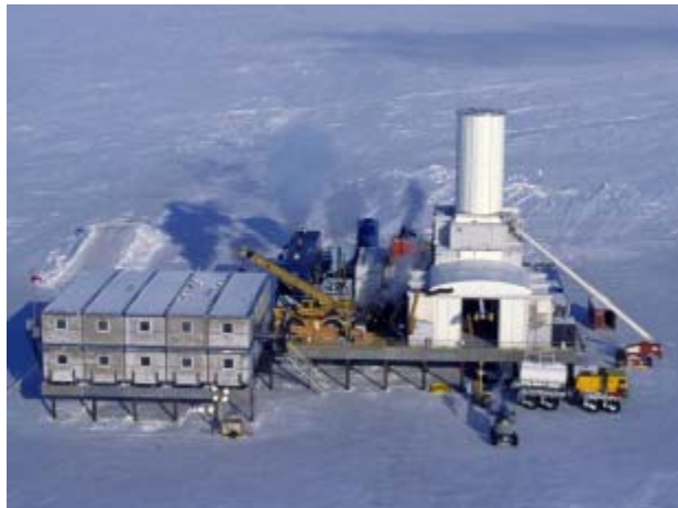
Figure A-5. Complete Camp Ready for Drilling
