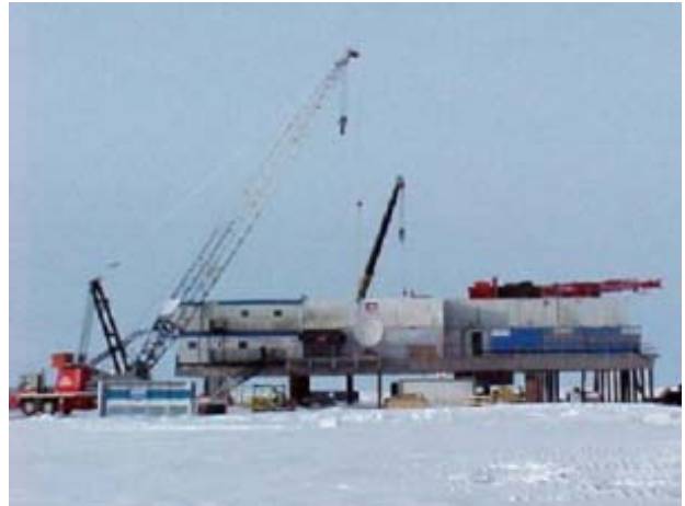
Figure A-4. Assembling the Platform
