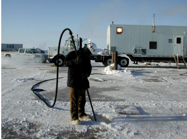
Figure A-13. Vacuuming Platform Leg Holes
