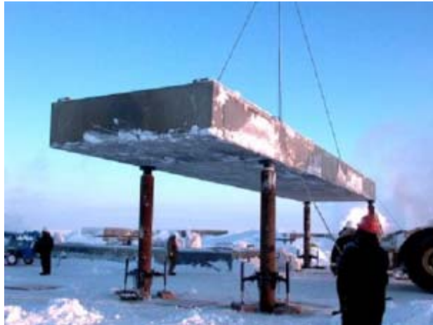
Figure A-3. Setting the First Platform Module
