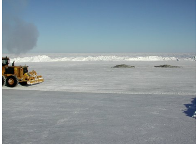
Figure A-14. Site after Demob & Remediation
