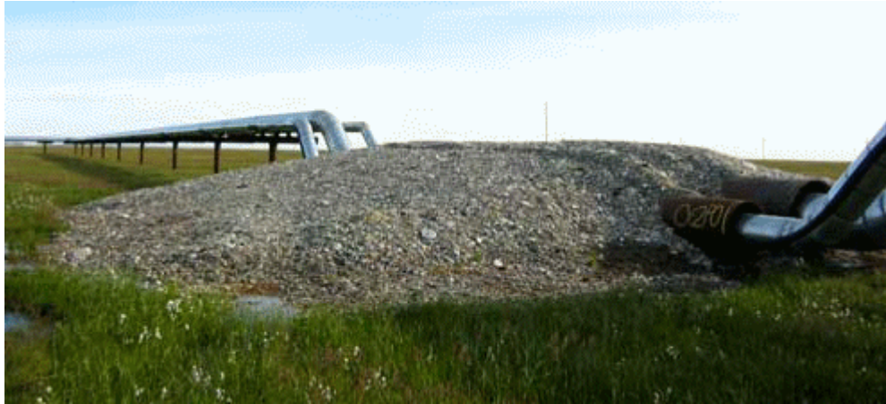
Figure 8. Gravel Ramp for Pipeline Crossing
