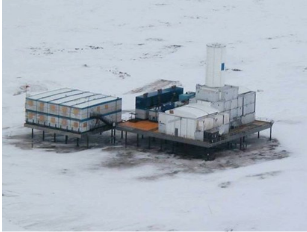
Figure A-7. Site at First Season Shutdown
