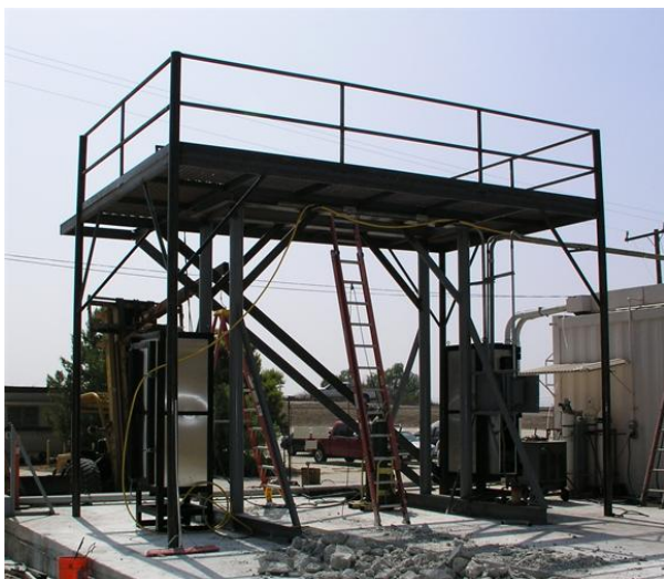
Figure 4. Reactor support framework before pilot plant assembly.
