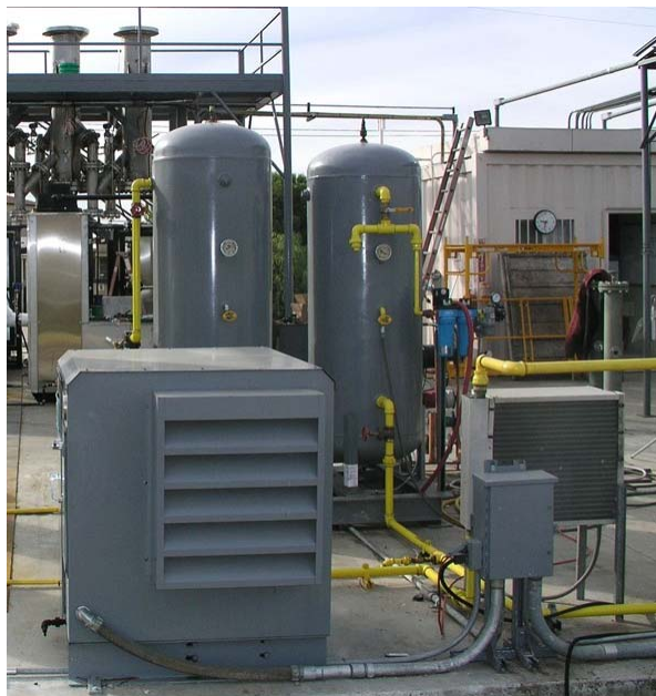
Figure 8. High-pressure air system assembly.
