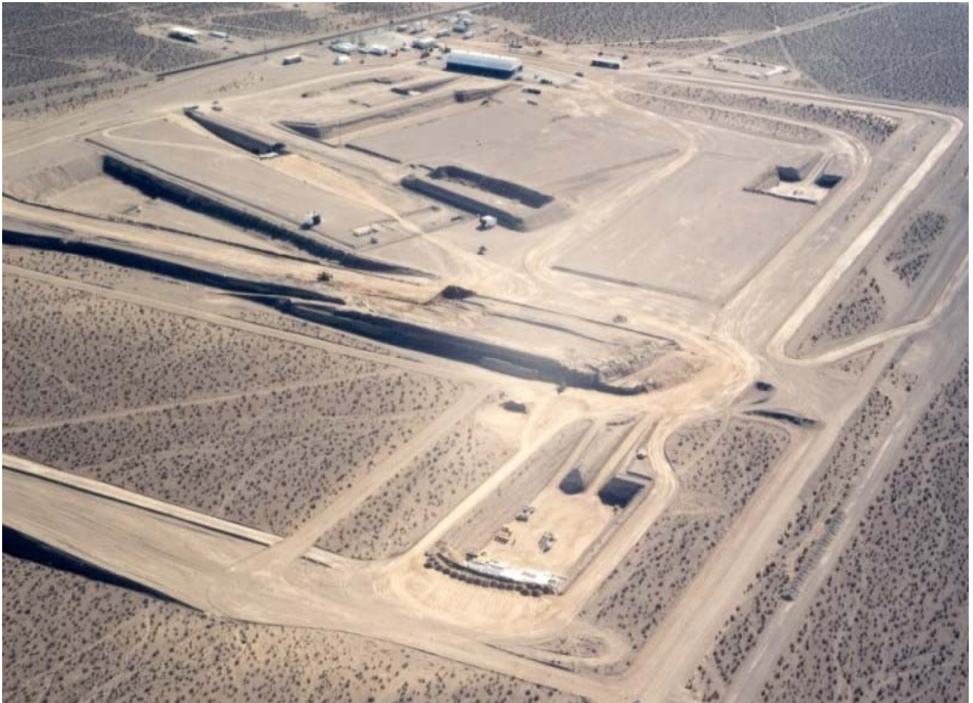
Area 5 Radioactive Waste Management Site, Nevada Test Site
