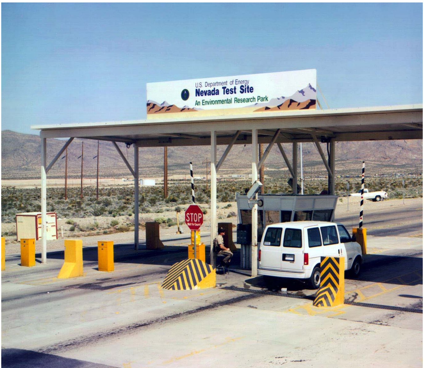
Gate 100 - Mercury, Nevada
