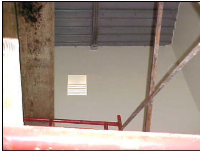
Figure 5. Passive as well as forced ventilation capability was installed in the upper section. Because of the thermal load requirement, a totally passive system was not possible.
