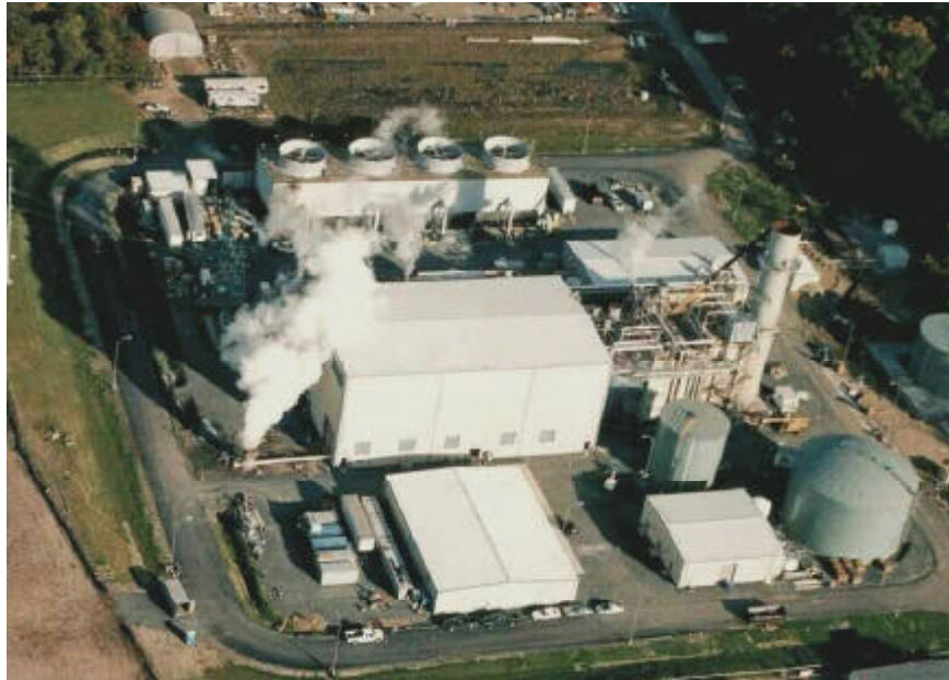
Figure 39: Photograph of the Combined Cycle Power Plant.
