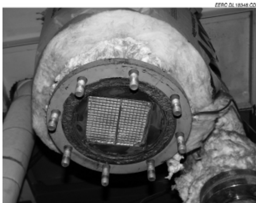
Figure 2-4 Photograph of the SCR Catalyst Following Test
