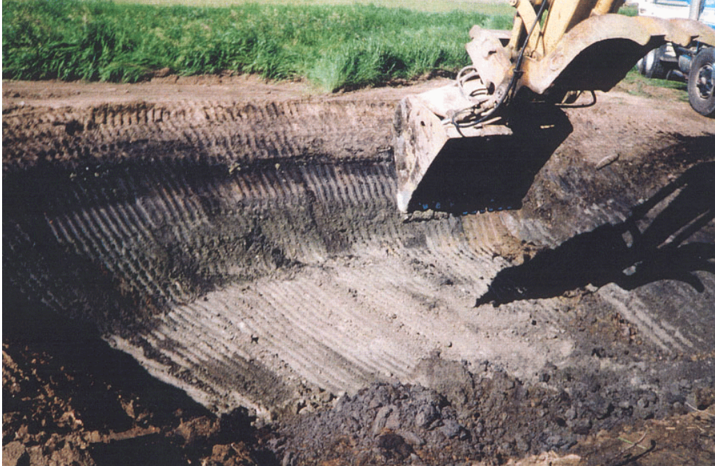
Photo 1. Amine contaminated soils (dark greenish grey) being excavated to utilize as treatment soils for laboratory and field based activities.
