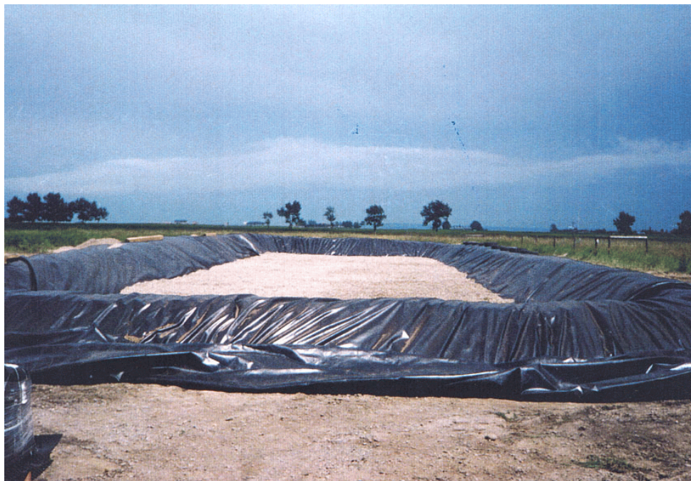
Photo 2. Biopile cell holding 40 mm drainage rock overlying the RPE 25 mil poly liner.
