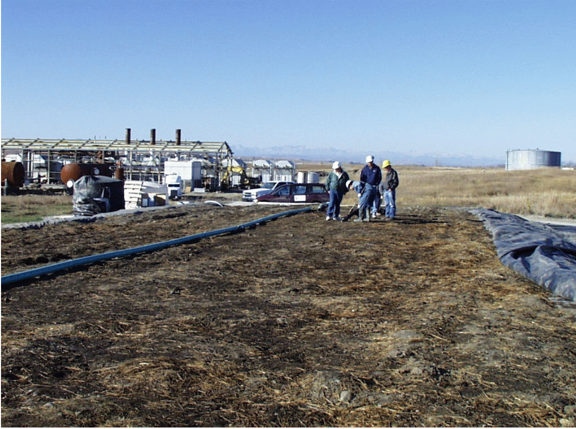
Photo 9. Biopile during sampling event. Note air vent running along the center of the pile and the cover trap pulled off to the north.
