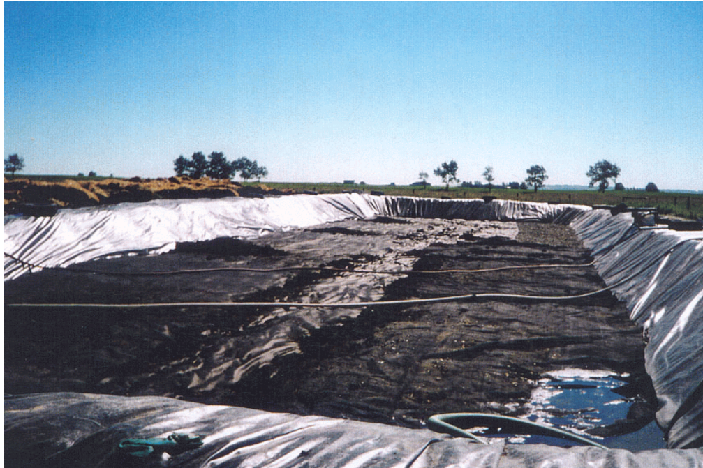
Photo 3. Biopile cell's filter fabric overlying the drainage rock.
