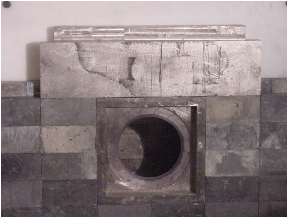
Figure 23. Lintel piece in place above the collar, showing the lead bricks carrying the load.
