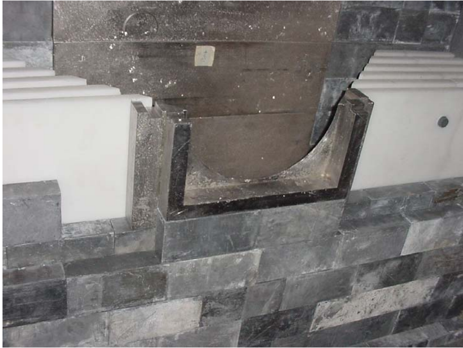
Figure 18. Lower half of the collar in position on the lead wall.
