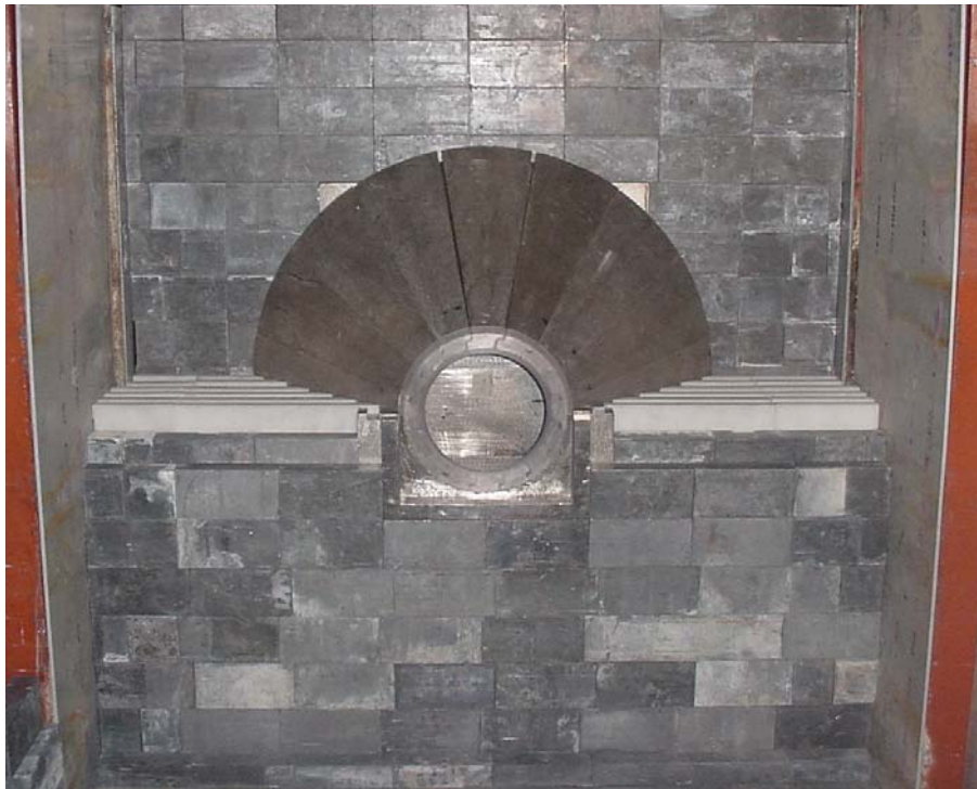
Figure 21. Top half of collimator staves in place.
