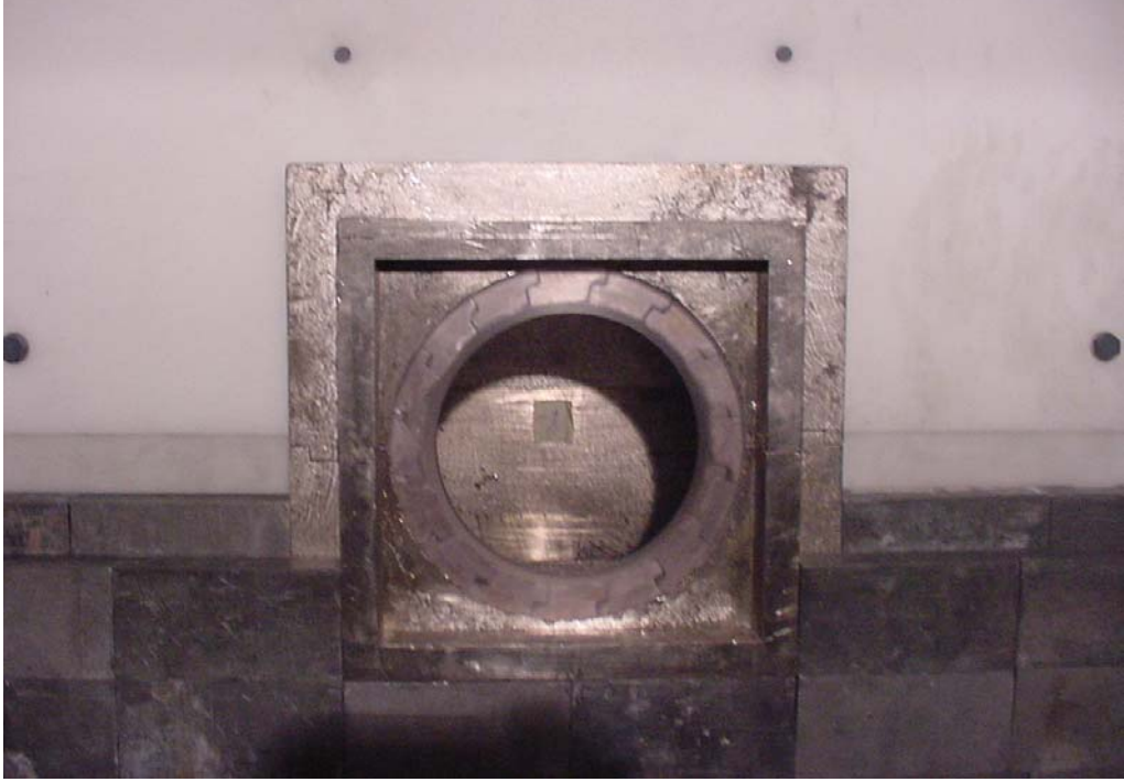
Figure 22. Upper half of collar in place.
