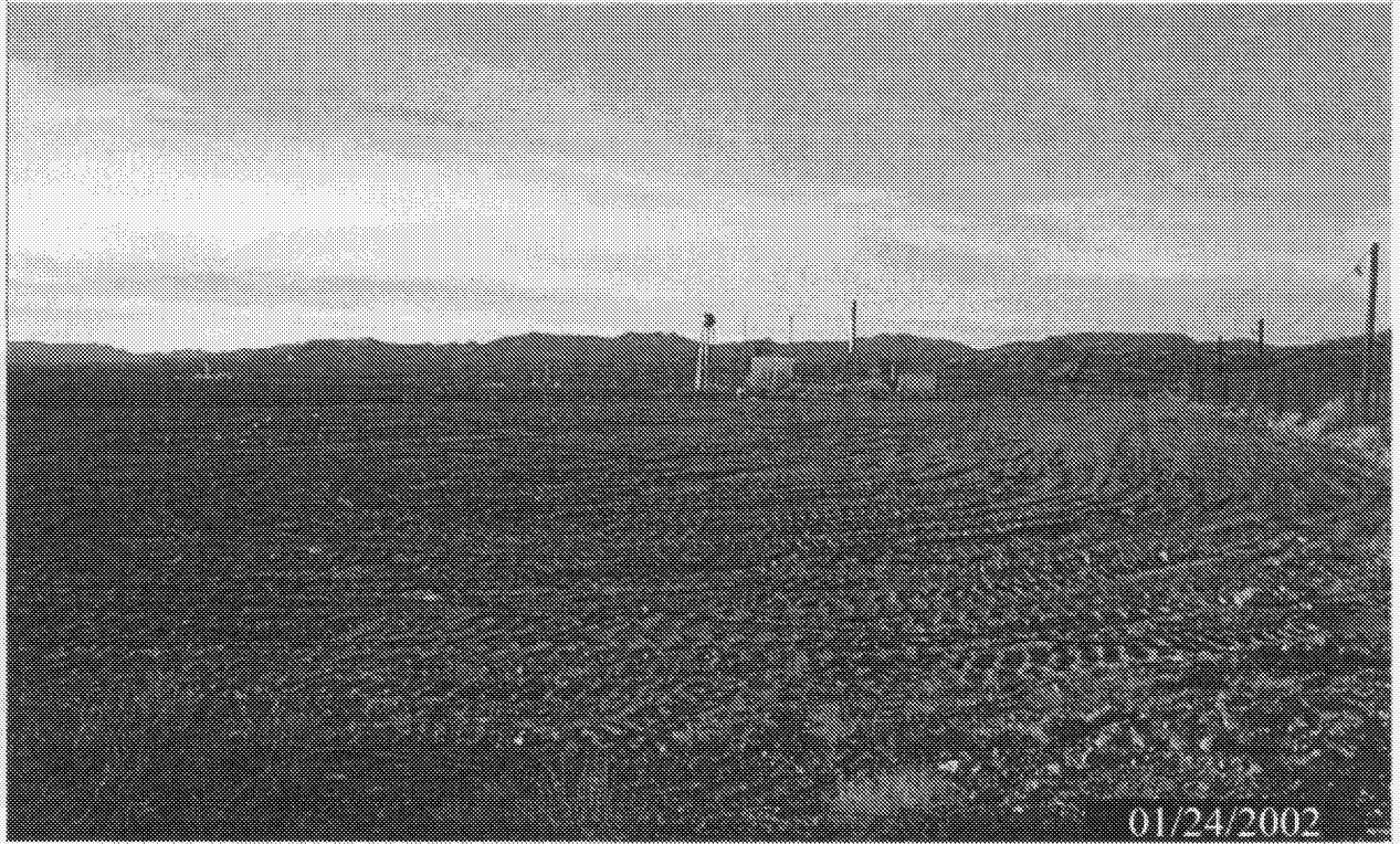
PHOTOGRAPH 4 - RMAD WEST TRENCH BERMS AFTER REMEDIATION
