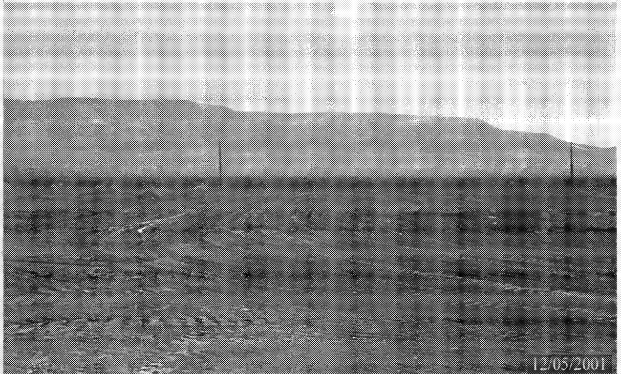
PHOTOGRAPH 2 - RMAD EAST TRESTLE AREA AFTER DEMOLITION
