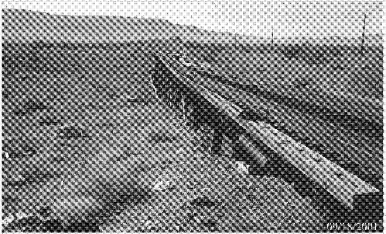
PHOTOGRAPH 1 - RMAD EAST TRESTLE AREA BEFORE DEMOLITION
