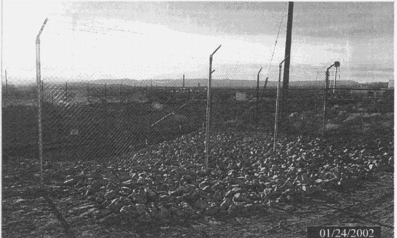
PHOTOGRAPH 10 - COMPLETION OF EROSION PROTECTION FOR SUBBASIN 4
