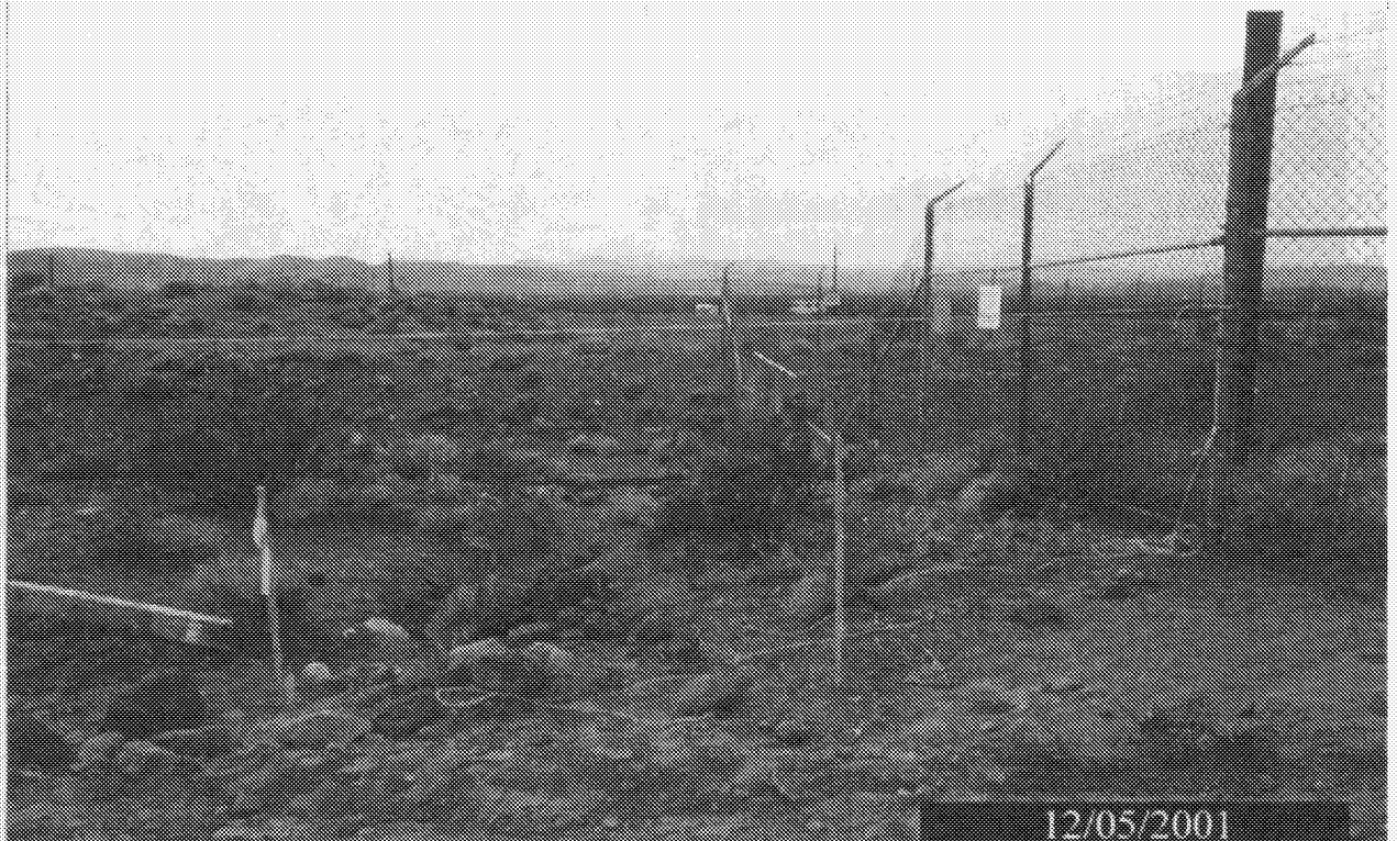
PHOTOGRAPH 6 - SUBBASIN 4 BEFORE EROSION PROTECTION INSTALLATION
