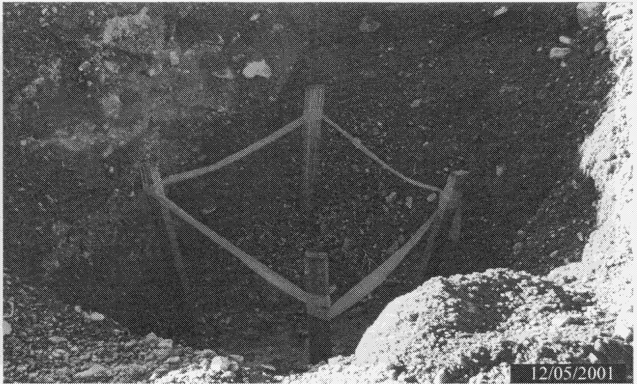
PHOTOGRAPH 11 - STRONTIUM-90 (Sr-90) IMPACTED SOIL EXCAVATION AREA
