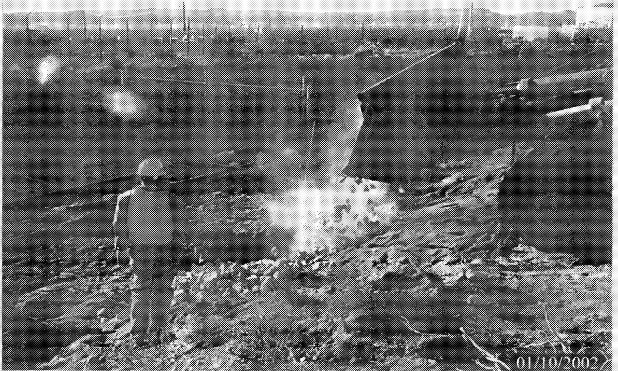
PHOTOGRAPH 8 - SUBBASIN 4 PLACEMENT OF RIP RAP ROCK MATERIAL
