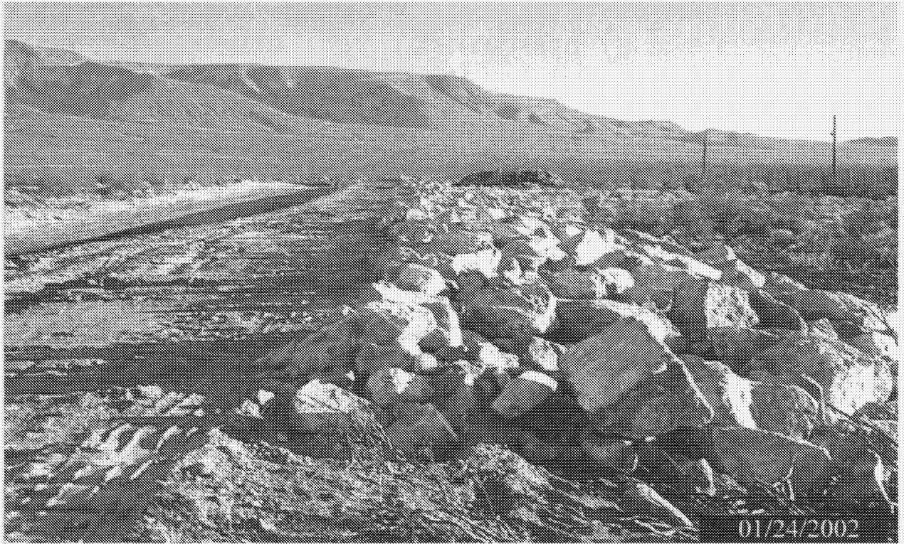
PHOTOGRAPH 13 - COMPLETION OF EROSION PROTECTION FOR SUBBASIN 5
