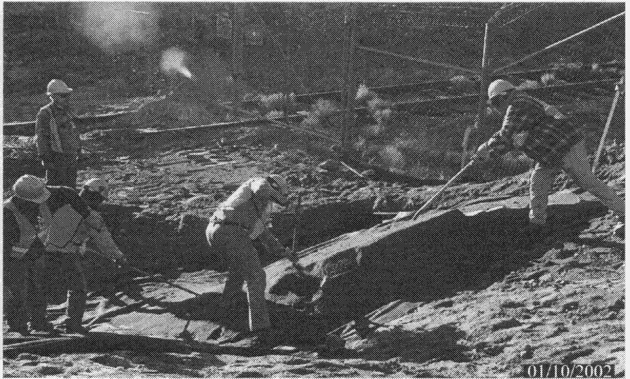
PHOTOGRAPH 7 - SUBBASIN 4 PLACEMENT OF SAND OVER GEOTEXTILE MATERIAL
