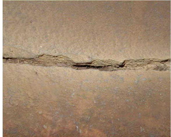
Figure 2. Camera's View of Bell and Spigot Joint Seam
