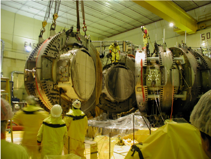
Initial segment removal
