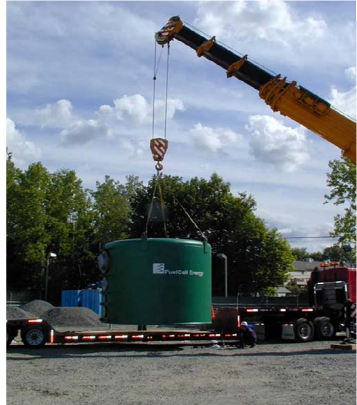
Figure 12. 4-STACK MODULE TRANSPORTATION HANDLING LOGISTICS VERIFIED: Loaded on a Double Drop Lowboy Using Standard Crane. Arrived at FCE Facility and Unloaded.
