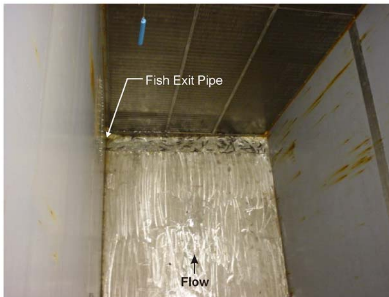
FIGURE 5-4 COLLECTION TANK BEING DRAINED AT THE END OF A TEST
