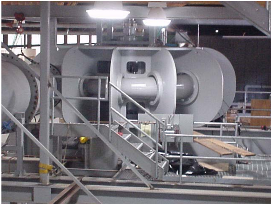
FIGURE 3-5 TURBINE SCROLL CASE
