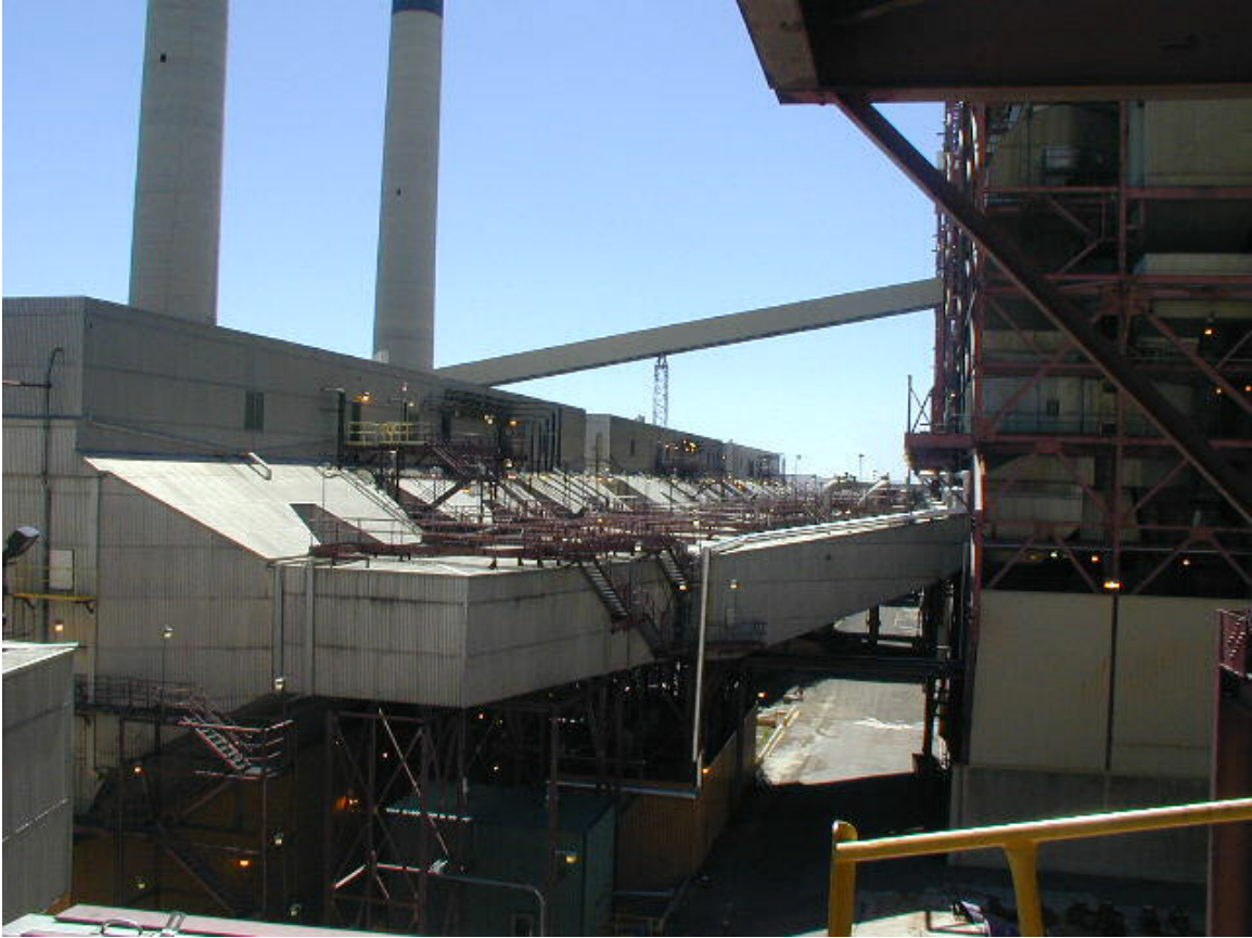
Figure 1: Inlet Duct and ESP at Potential Long-Term Site
