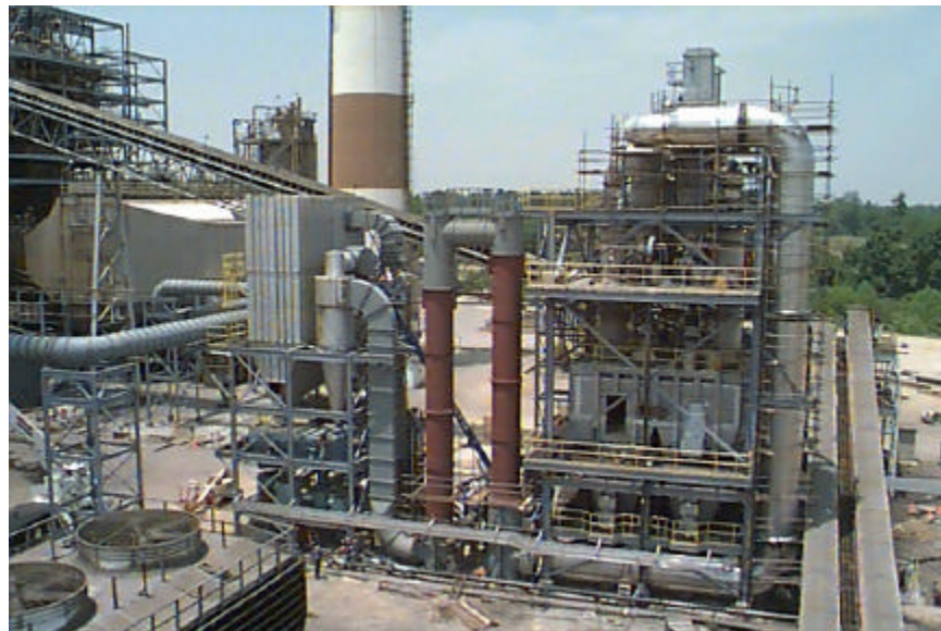
Figure 7.2-1: Carbon Burn Out™ Installation
