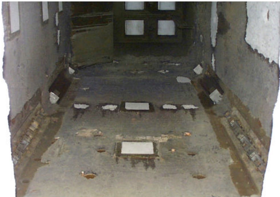
Figure 6.3-5: Inside View of the North Wall of the BSF.
