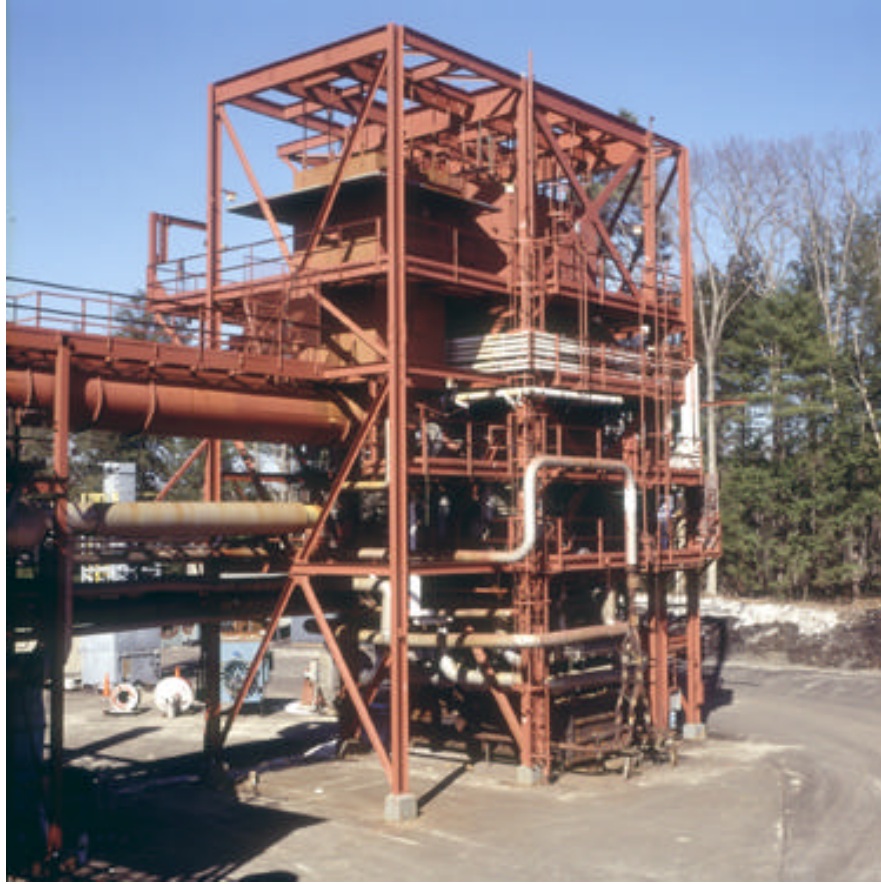
Figure 6.2-1: Boiler Simulation Facility.
