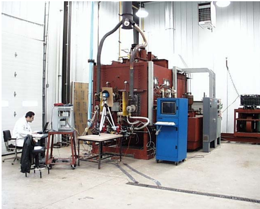
Figure 21. THERMAL IMAGING CONTROL OF THE GTI HEAT TREAT FURNACE
