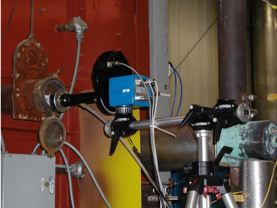
Figure 17. FURNACE AND TIS SET-UP AND TIS COMPONENTS
