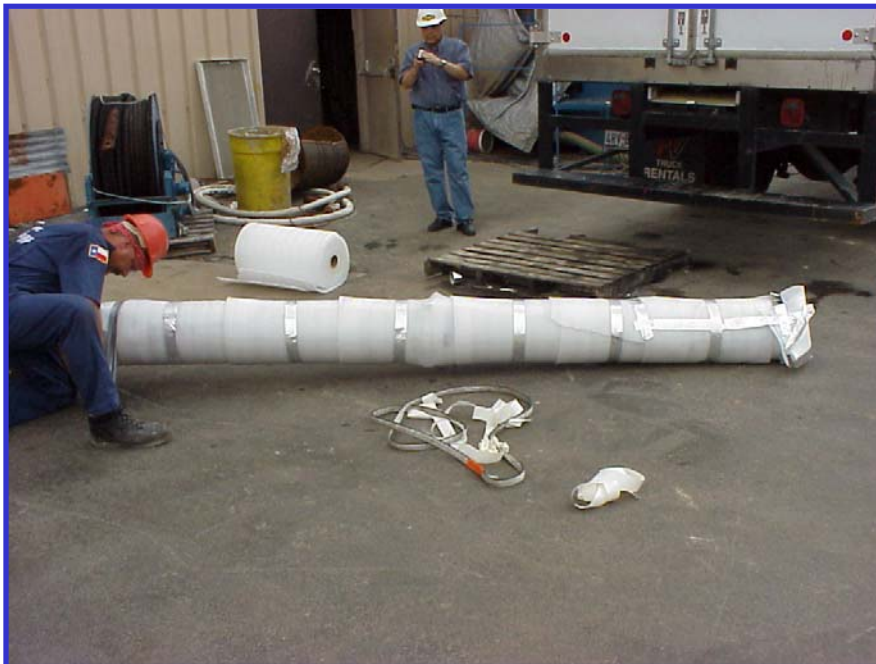
Figure 29: Frozen Core Preparation Before Coring Operation (Cont'd)
