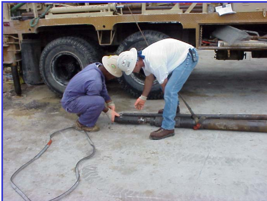
Figure 33: Coring Tools Preparation
