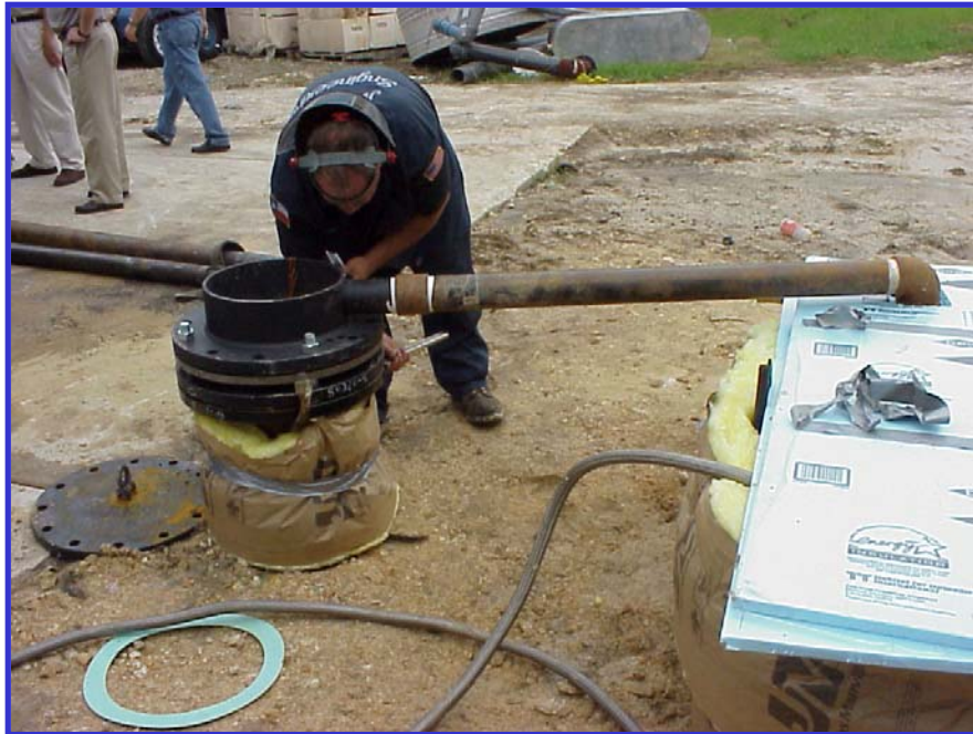
Figure 32: Wellhead Preparation Before Coring
