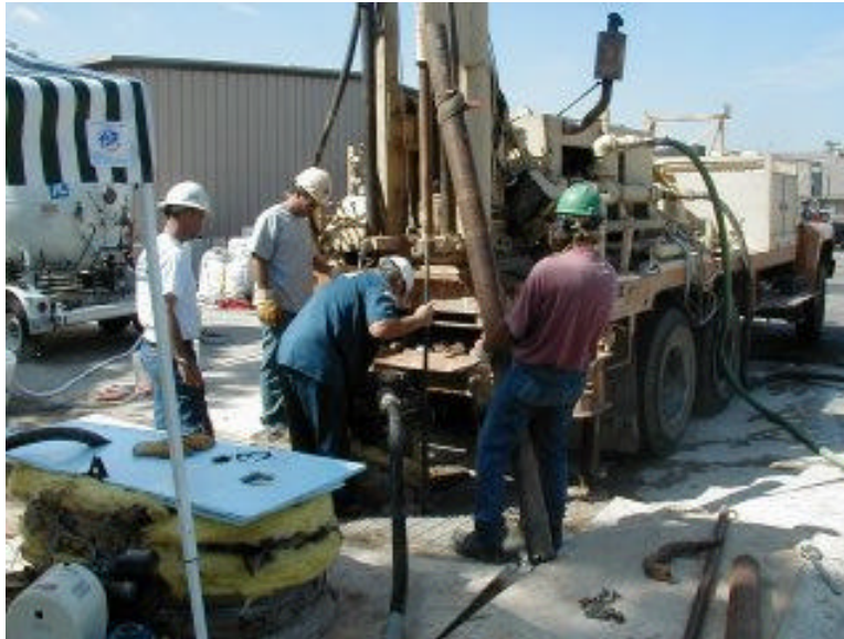
Figure 10. Environmental Coring Rig
