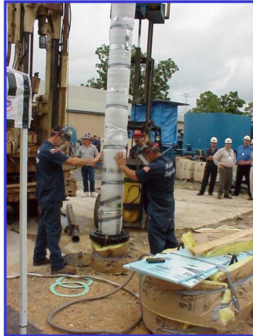
Figure 30: Frozen Core Placement in the Well to Be Cored
