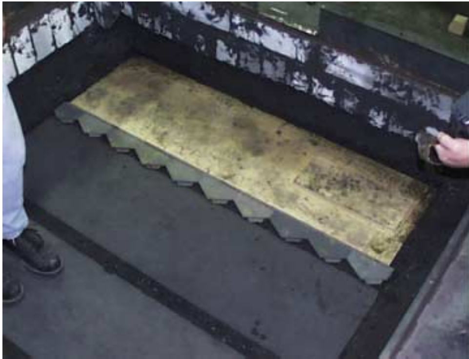
Figure 7 - Installation of Drained Edge Tiles
