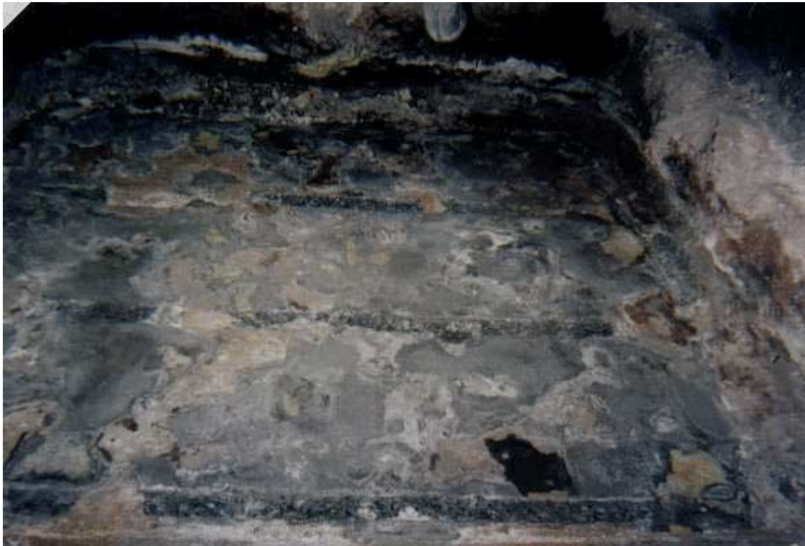
Figure 13 – Pilot Cell 1 Showing Erosion of Cathode and Rammed Toe
