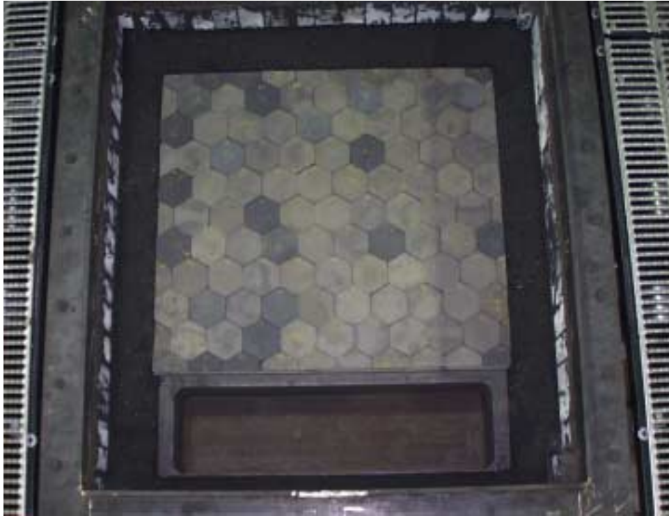
Figure 9 - Overview of Completed Tile Installation
