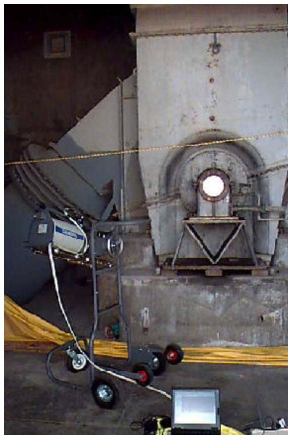
Figure 5-1. In situ measurement of Fan No. 3
