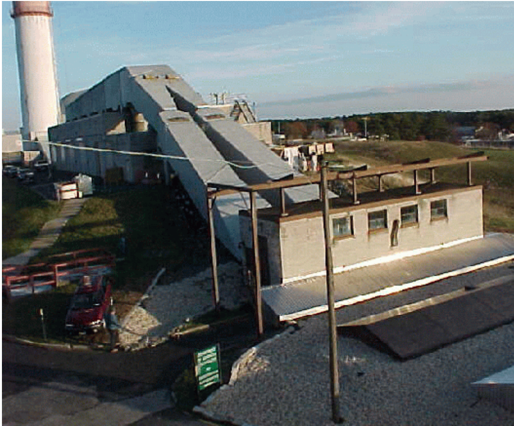
Figure 1 Above ground ducts and Fan House at the BNL BGRR
