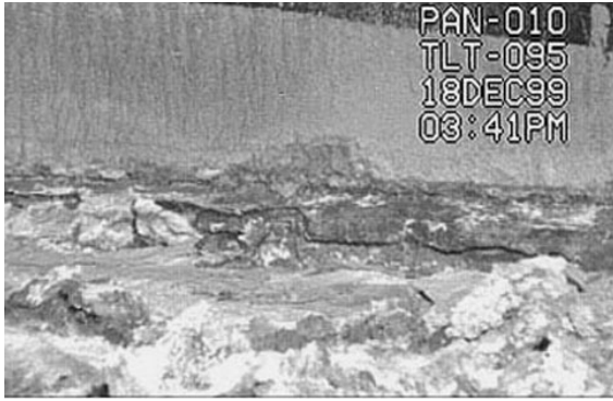
Figure 4.1 Tank Wall Waste Retention During Transfer 1
