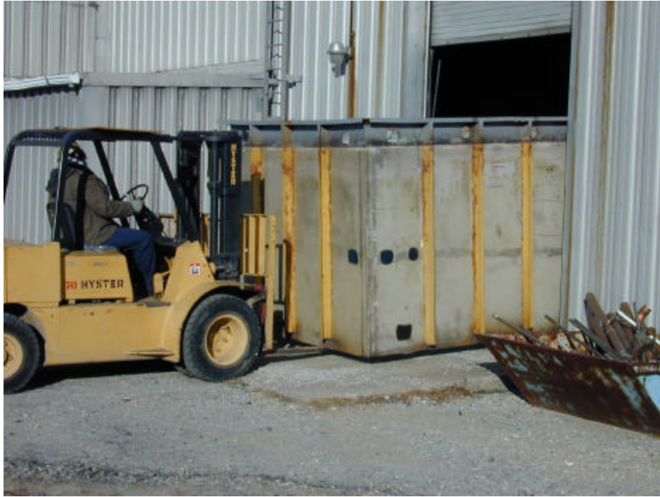
Figure 24 Moving the tank's top half out the roll-up door.
