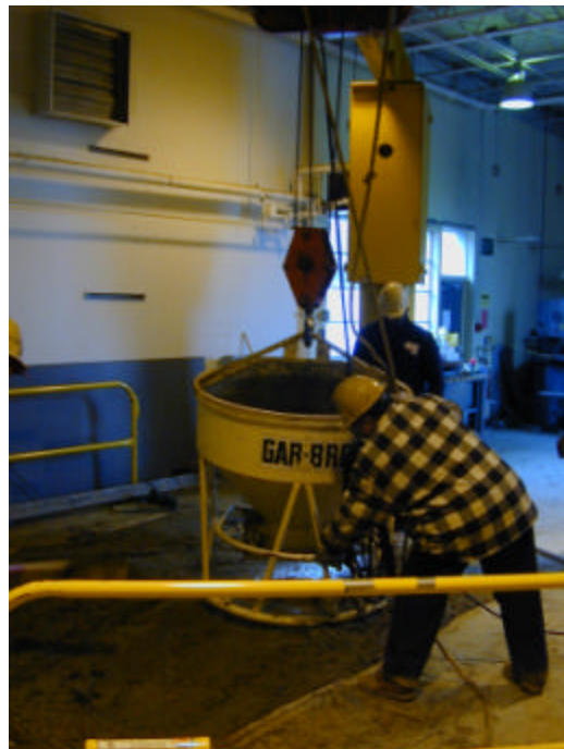
Figure 30 Installing the concrete cap.
