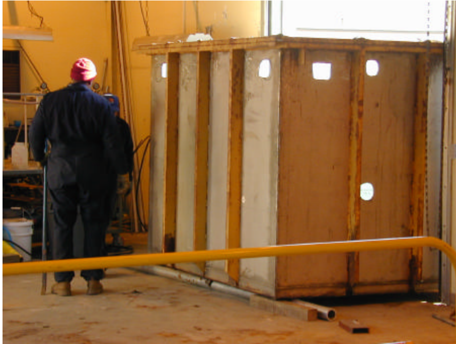
Figure 26 Moving the lower half of the tank out the door.
