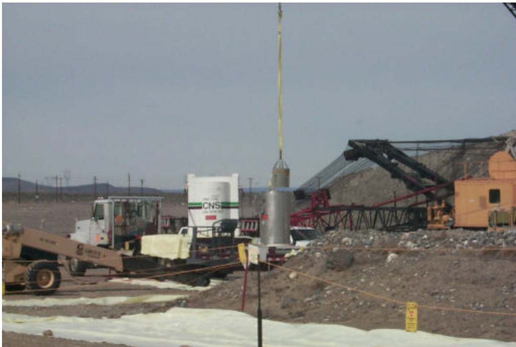
Figure 20 Liner being unloaded at the Hanford DOE disposal facility.
