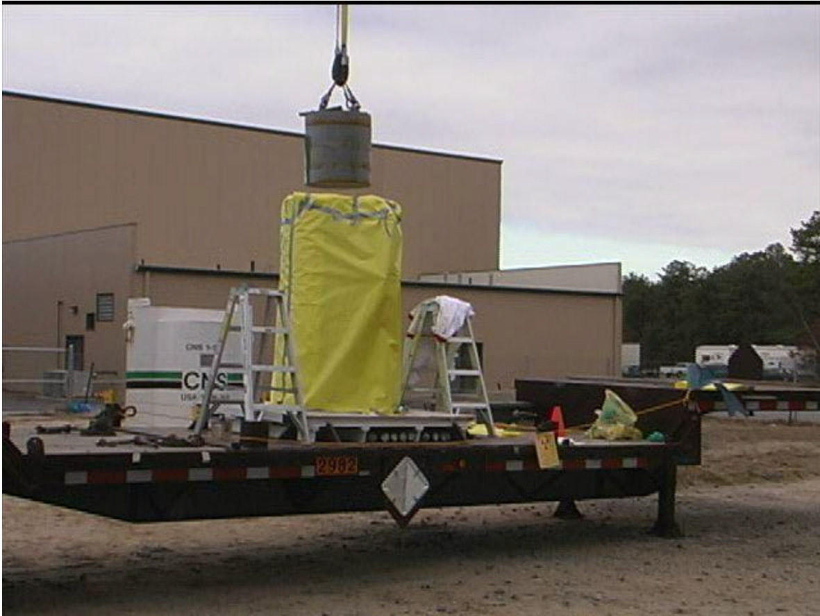
Figure 19 Liner being lowered into shipping cask.
