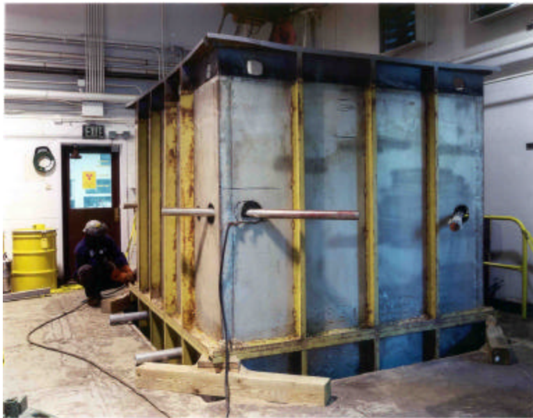
Figure 23 Plasma torch cutting along the original weld seam.
