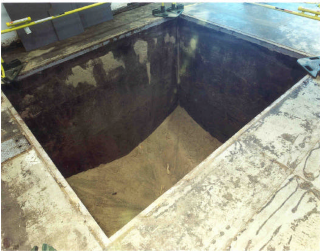
Figure 28 The empty pool pit, with original tank backfill sand.
