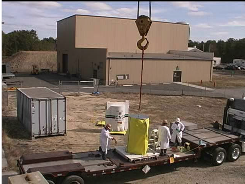
Figure 13 Shipping cask preparation – Removing the contamination seal cover. (Cask was wrapped because low levels of contamination were found under impact cover.)
