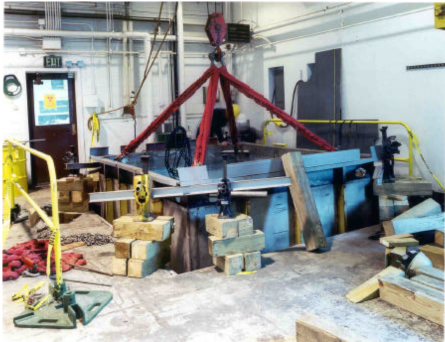
Figure 21 The liner lifted slowly from its installed position.
