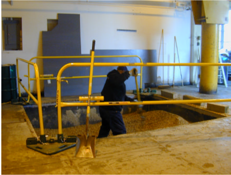
Figure 29 Spreading and tamping the gravel backfill.
