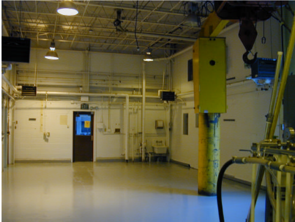
Figure 31 The finished product, an empty room with a crane.
