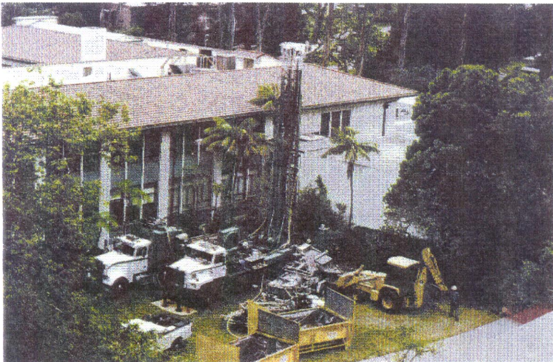
Figure 24. (bottom) Drilling rig in operation at UCSB adjacent to Webb Hall. Two deep (~75 m) boreholes were made.
