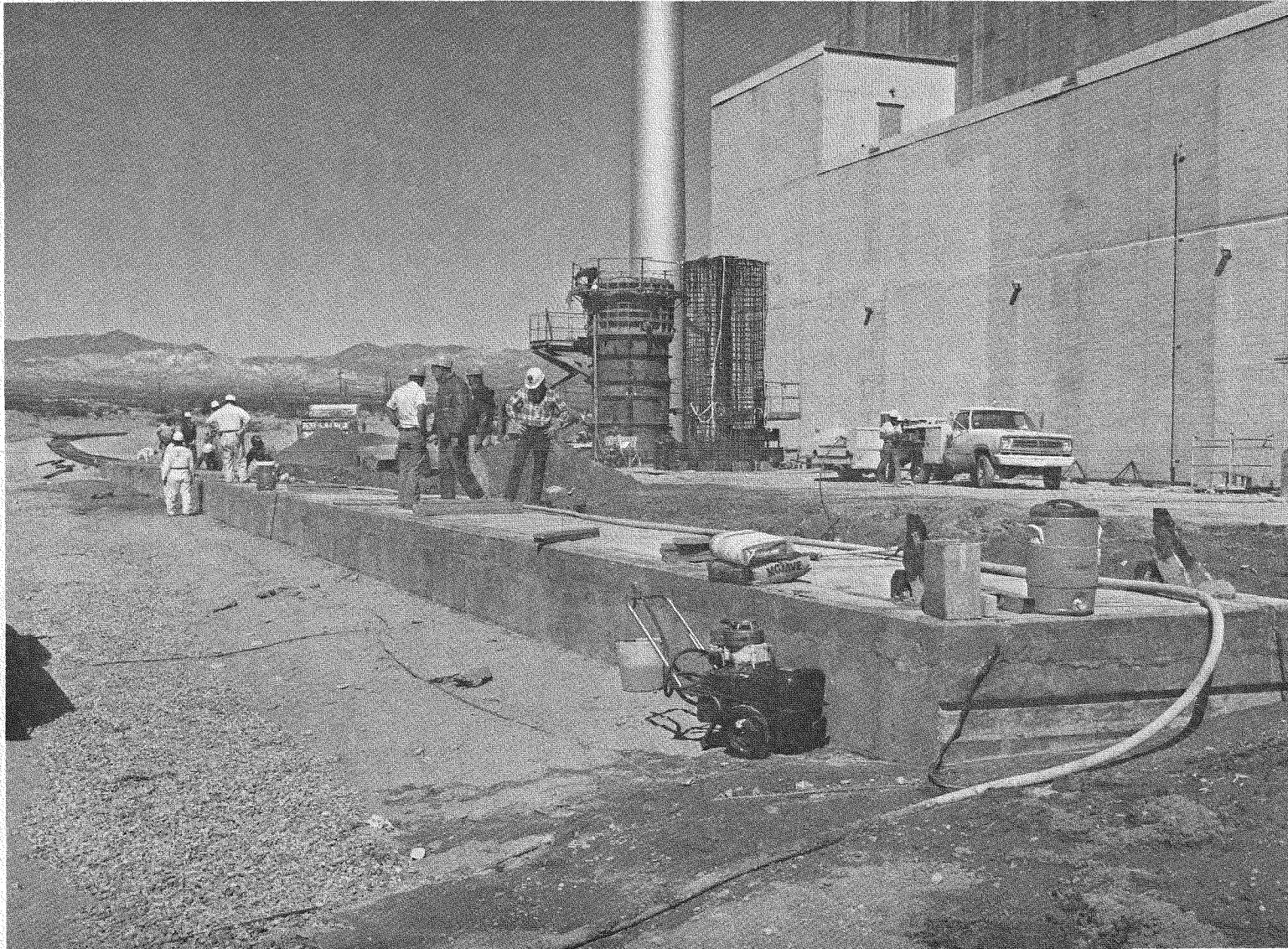
Figure 16. SSC and Drywell Storage Area Construction
