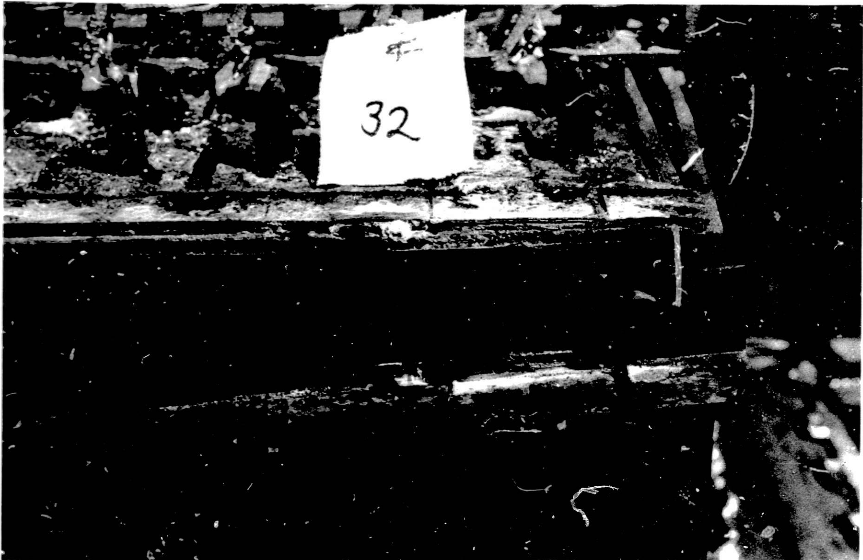
Fig. V-5. Evidence of Reaction Similar to that Observed at Cell 27/28 (analysis of metallic material from this area showed mostly iron and aluminum)
