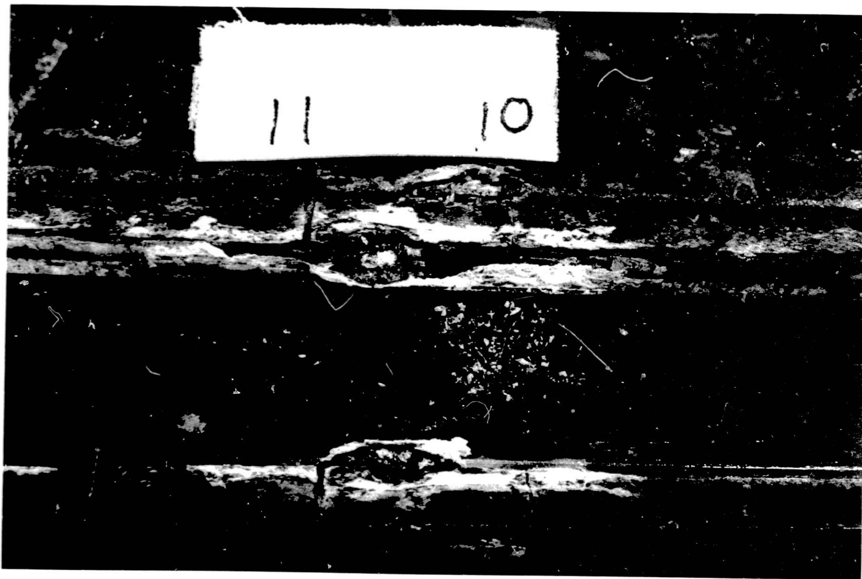
Fig. V-9. Badly Corroded Area at Top Edge of Cells 10/11 (Similar to that observed at Cells 27/28 and 32/33. Part of the corroded material is adhering to the tray angle.)
