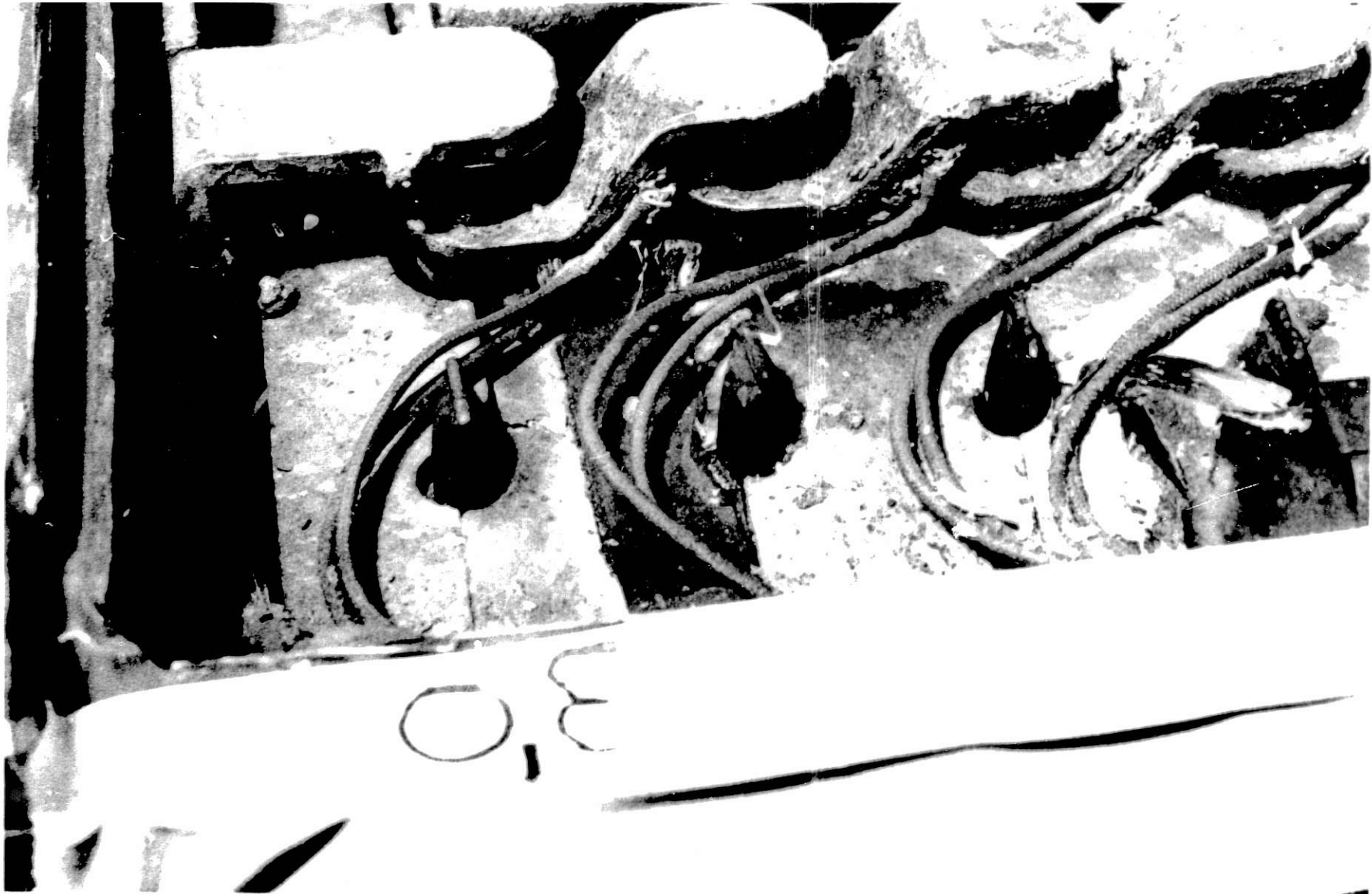
Fig. V-4. Cross-over Strap in Region of Cell 29 Fill Tube (evidence of arcing or burnout apparent at contact point)
