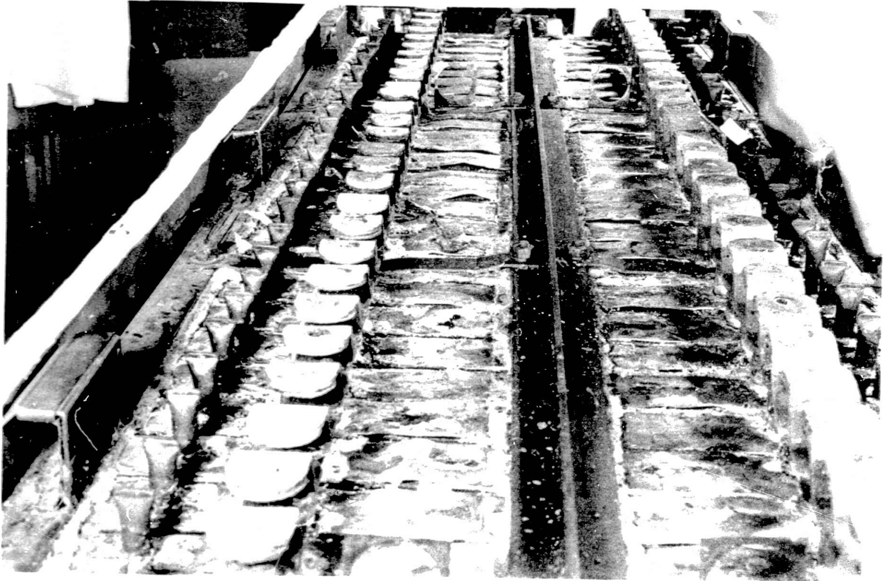
Fig. V-7. Top View of Module (The cell top insulation has been removed and evidence of electrolytic corrosion and braze melting is visible. In many areas, metallic bridges were formed between cells across the top of the mica insulation.)
